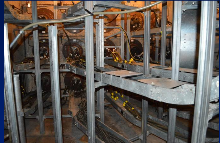
Zion U2 Cable Spreading Room
