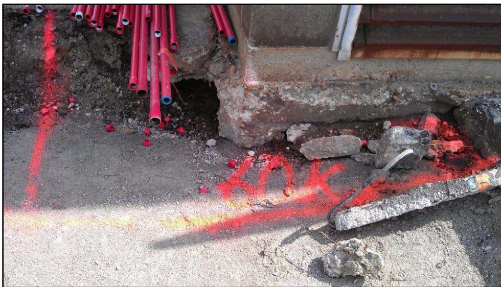
Figure 18-17 NW Corner of Building 215 (Elevated Area)
