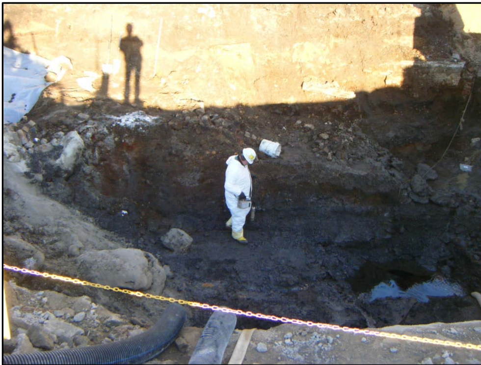
Figure 18-9 Photograph (7) of SU12 North of Vertical Pipe Stand (East View)
