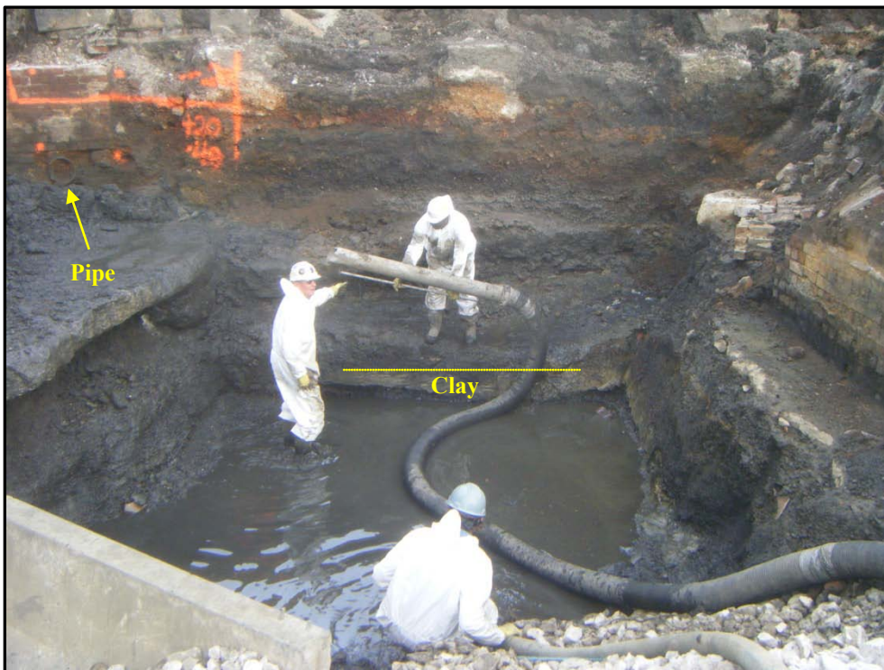
Figure 18-6 Photograph (4) of SU12 South of Vertical Pipe Stand (East View)
