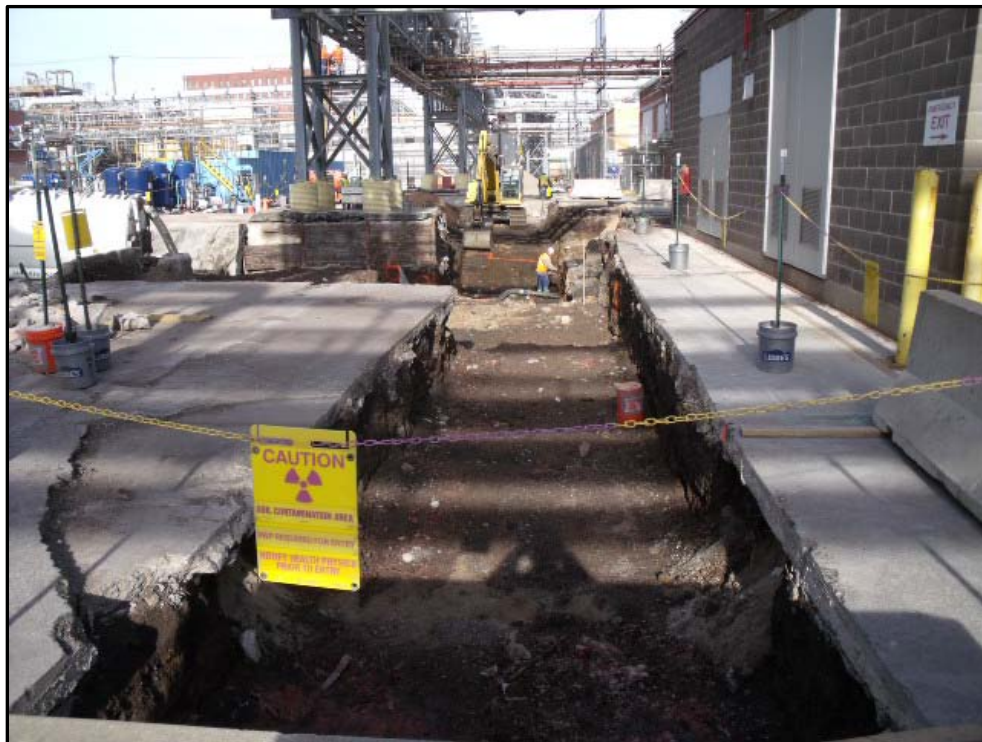
Figure 18-3 Photograph (1) of SU12 Looking along 7 th Street Alley (North View)
