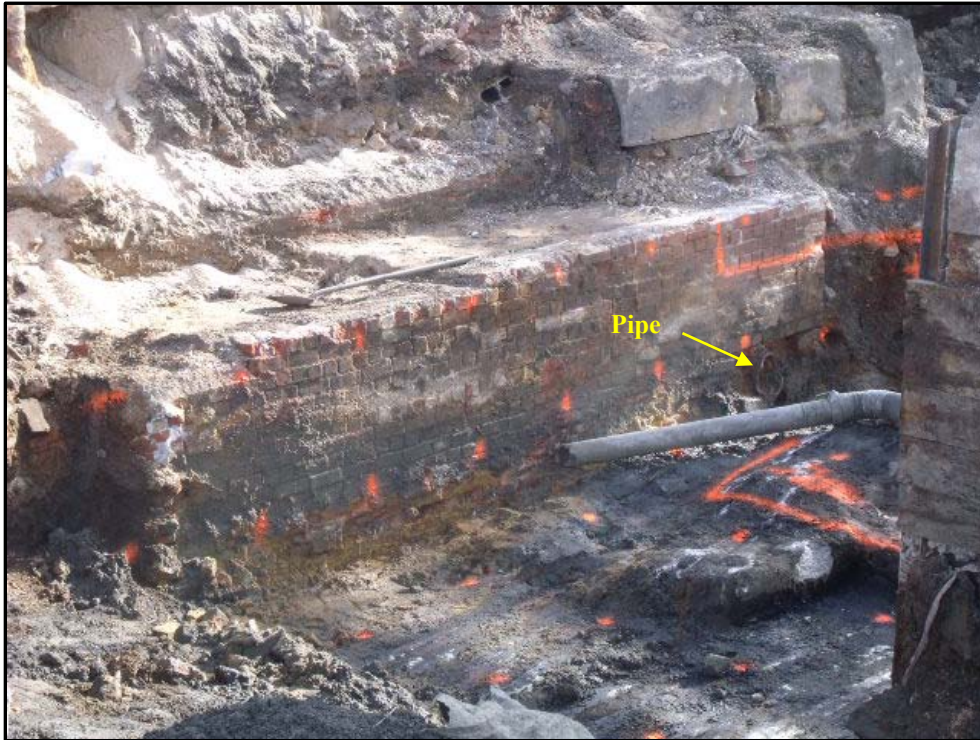
Figure 18-7 Photograph (5) of SU12 Subsurface Structures (Southeast View)
