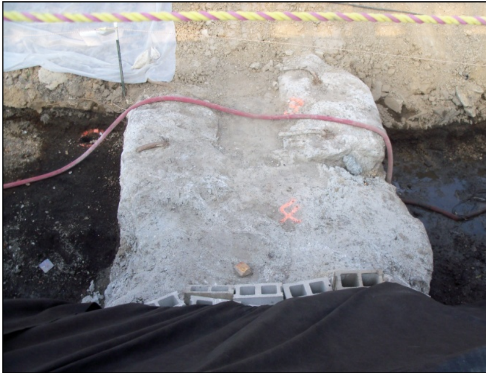
Figure 10-4 Photograph of Legacy Concrete in SU04
