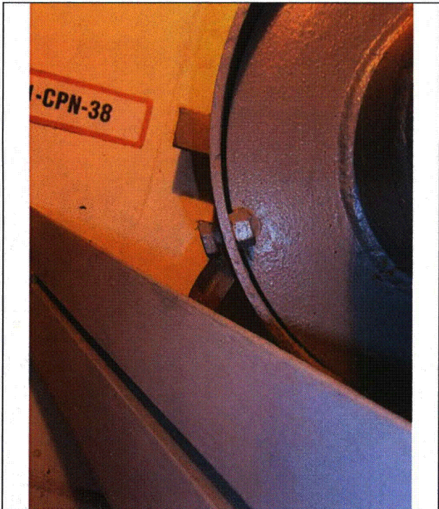
Note: Backed out bolt on 1-CPN-38 (P3280102)
