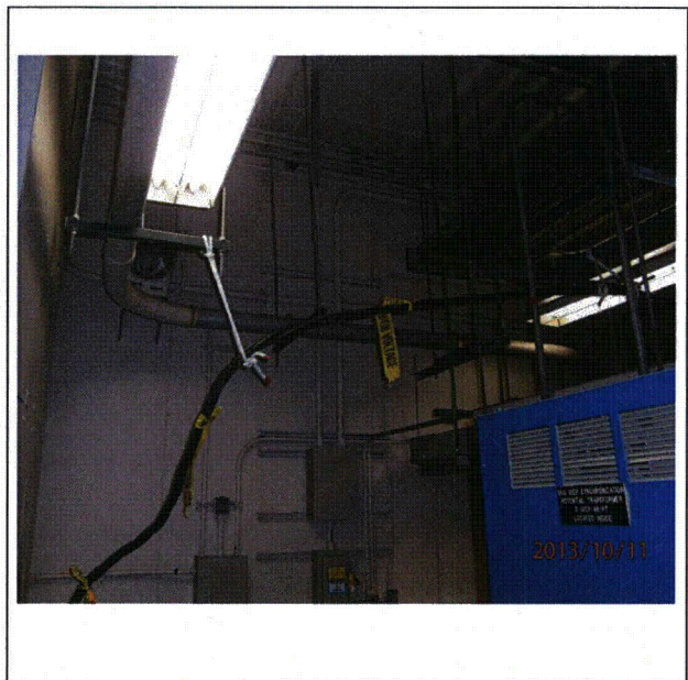
Note: (PA110630) Temporary power for Unit 2 Cycle 21 refueling outage.
