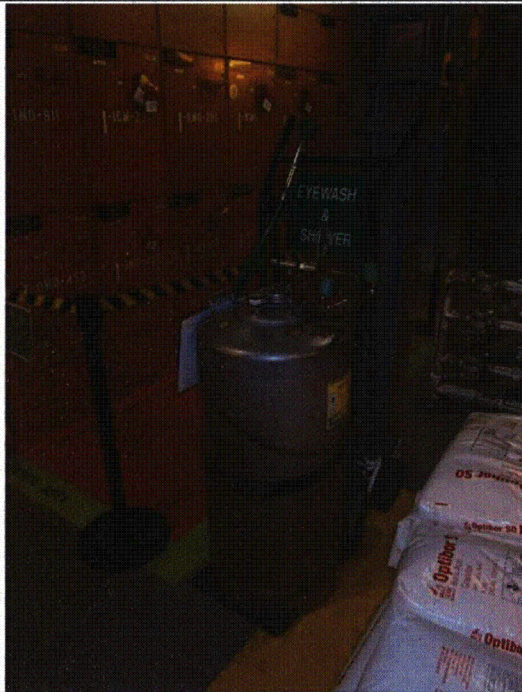
Note: Eyewash and shower station properly tied off and restrained (P4050294)
