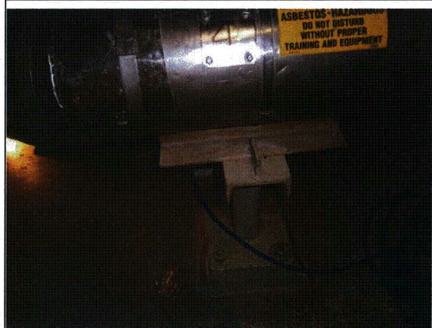
Note: Cord staged for Radiation Protection remote coverage for the Unit 1 Cycle 25 Outage (P4010155)
