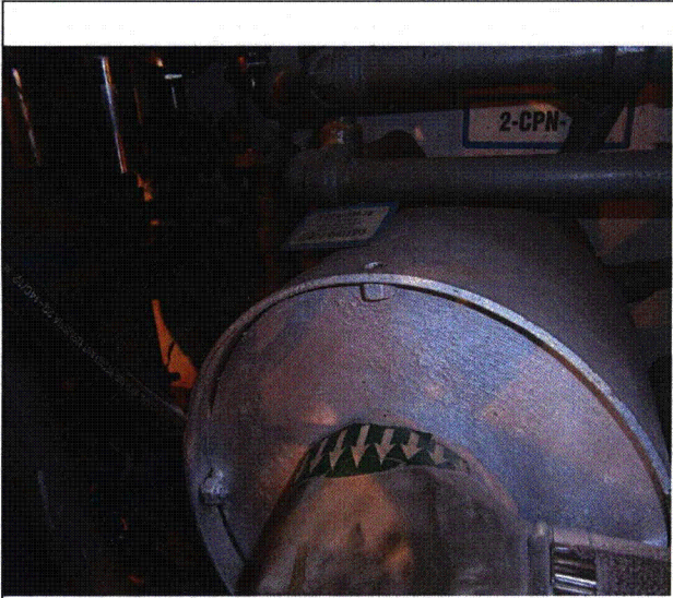
Note: (PA-040555) 2-CPN-79 missing bolts. (See Comments Above)
