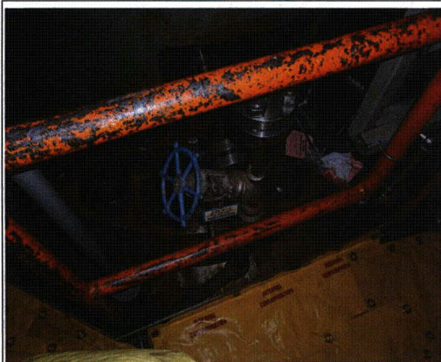
Note: (PA-040454) Lead shielding and plastic and maintenance in use equipment hung for Unit 2 Cycle 21 Outage
