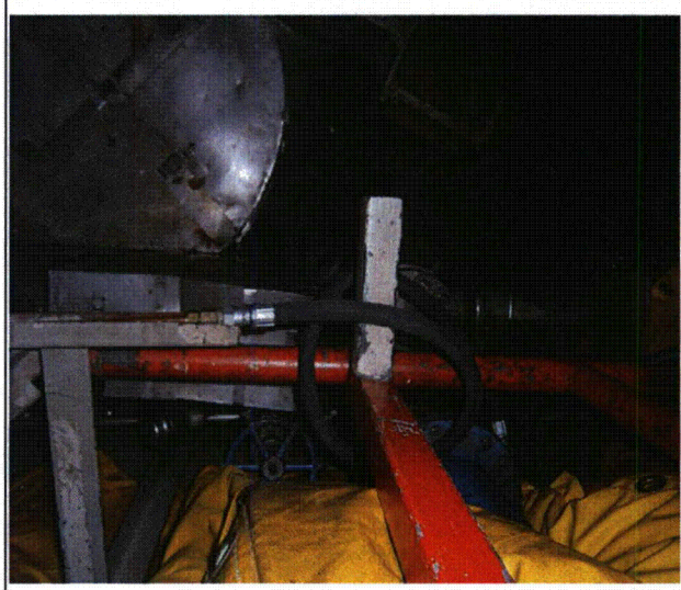
Note: (PA-040458) Lead shielding hung for Unit 2 Cycle 21 Outage.
