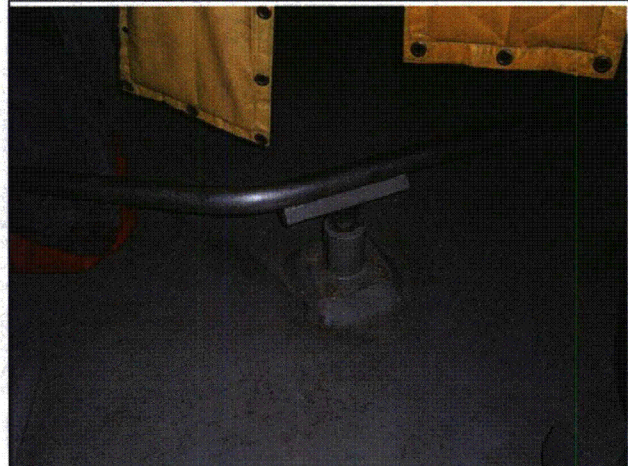
Note: Lead shielding hung for Unit 1 Cycle 25 Outage(P4010133)
