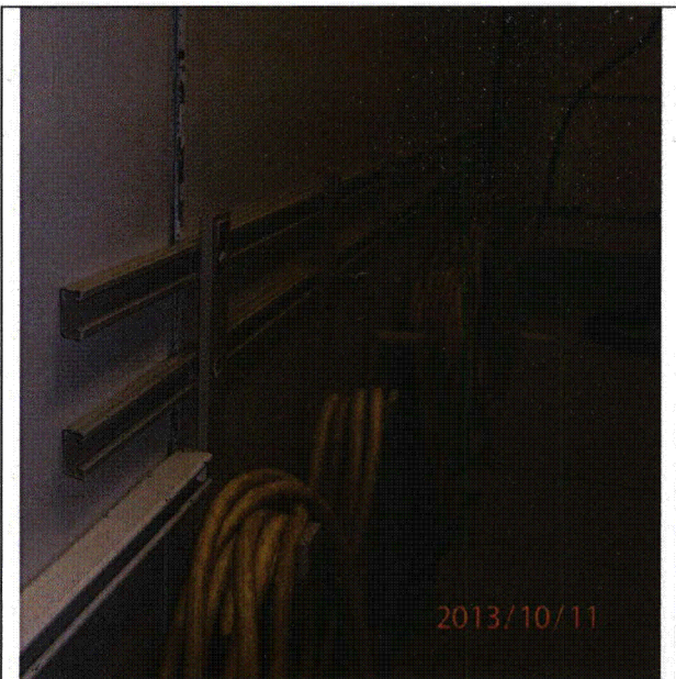
Note: (PA110628) Missing eyebolt in one hook, not a seismic concern.
