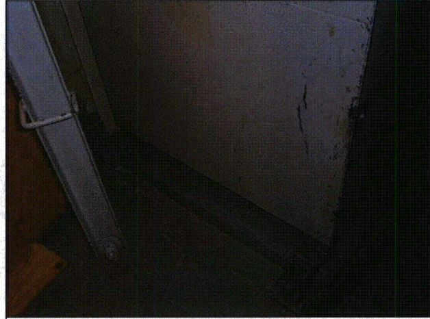
Note: Lead shielding hung for Unit 1 Cycle 25 Outage (P4010130)
