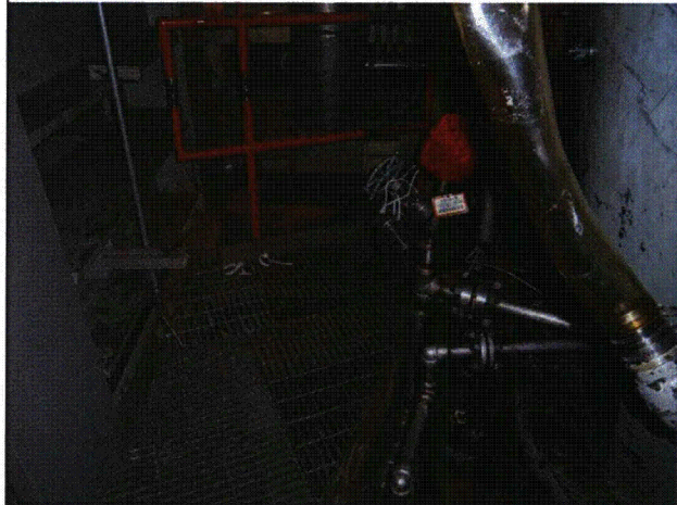
Note: Red FME cover in place for the Unit 1 Cycle 25 Outage (P5081552)
