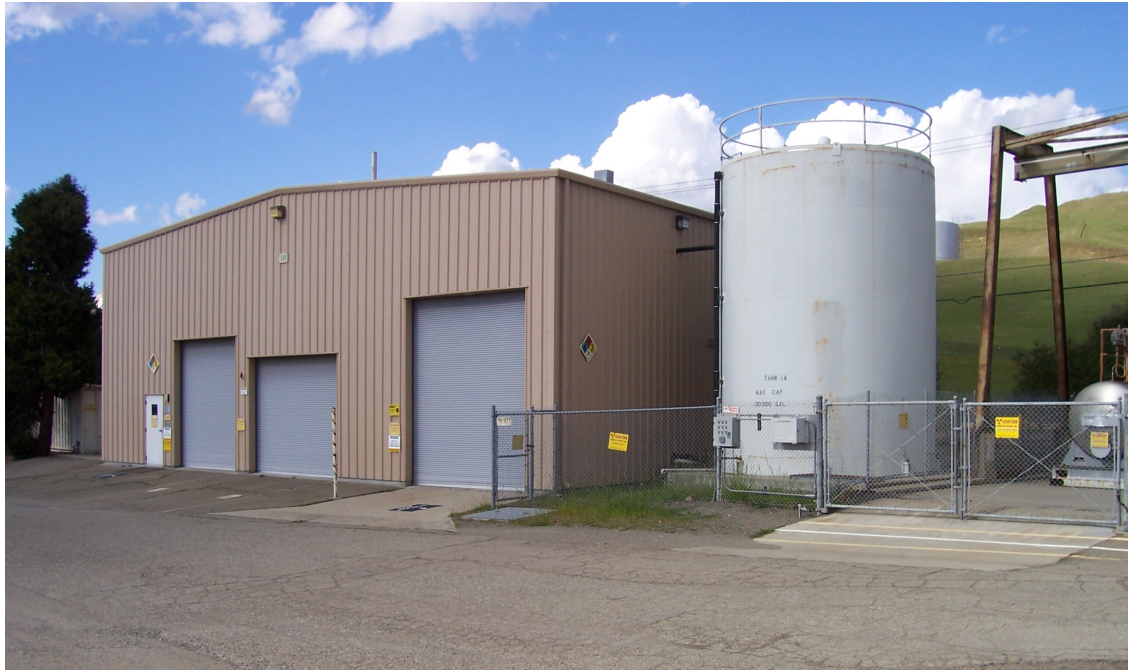
Photo 1.6 – WEP view of southside and 30,000 gallon tank
