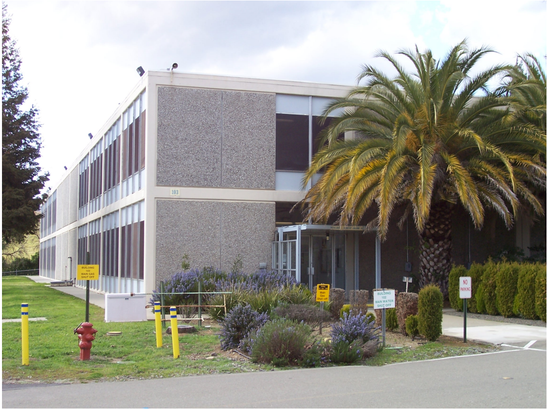
Photo 1.3 – Building 103 southeast corner view
