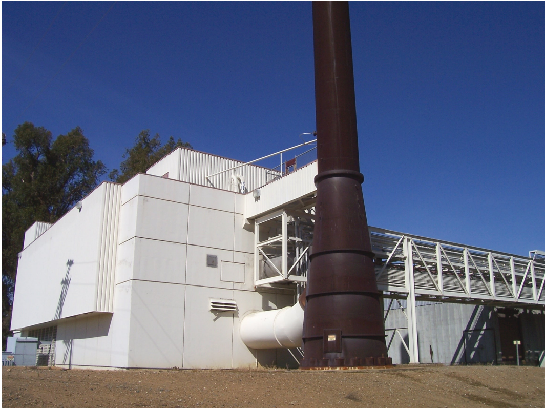
Photo 1.2 – Building 102A east side
