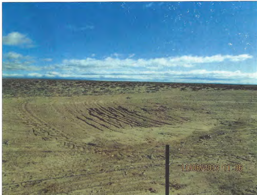
Photo Number 25: This depicts some rilling on the newly reclaimed area east of the pond diversion ditch. These rills will need to be repaired.
