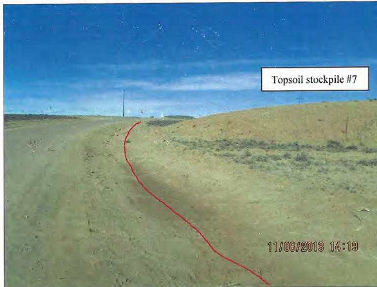
Photo Number 13: This depicts the west edge of topsoil stockpile #7. This stockpile is immediately adjacent to the road that leads to MU1 from the Plant Site. This view is looking north. The road ditch indicated with a red line in this photo also (currently) functions as the stockpile's toe-ditch. This is an unacceptable geometry and must be remedied immediately. The topsoil stockpile must have a unique and wholly separate toe ditch from the road's ditch.
