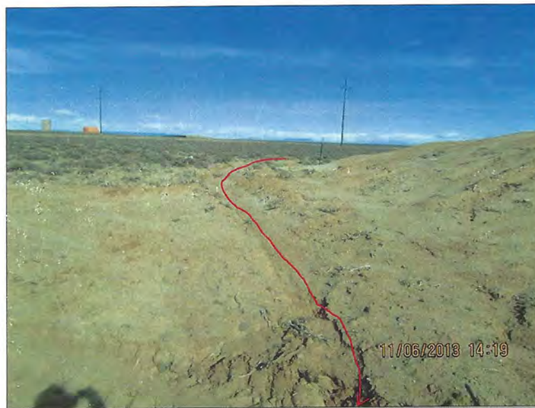
Photo Number 14: This depicts the northwest corner of topsoil stockpile #7. The portion of the stockpile's toe ditch that runs along the north edge of the stockpile is indicated here with a red line. The red arrow (bottom of the photo) indicates where that toe ditch empties (via rills) into the road's borrow ditch. As indicated in the caption for Photo Number 13, above, this is unacceptable and must be redesigned. Topsoil will be lost to the road's ditch if this is left as-is.
