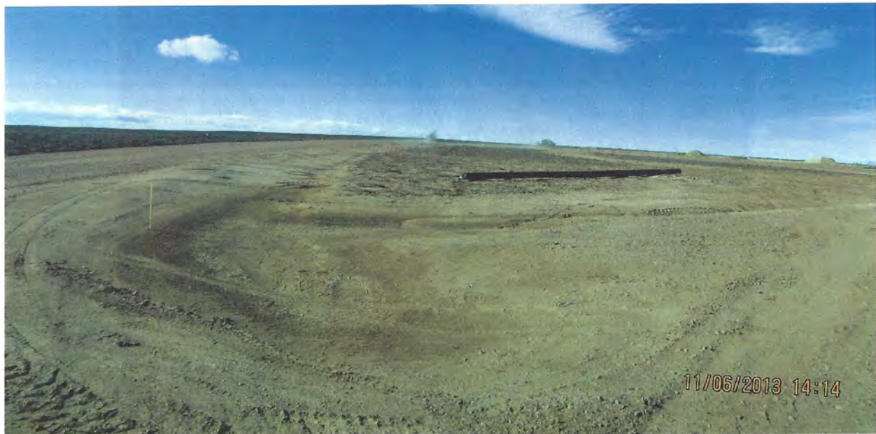
Photo Number 30: This is looking west at the intersection between the fire access road to the Plant Site with the main access route to the Plant Site. A culvert will need to be installed under the fire access route at this location due to the accumulation of materials indicated by the red oval.
