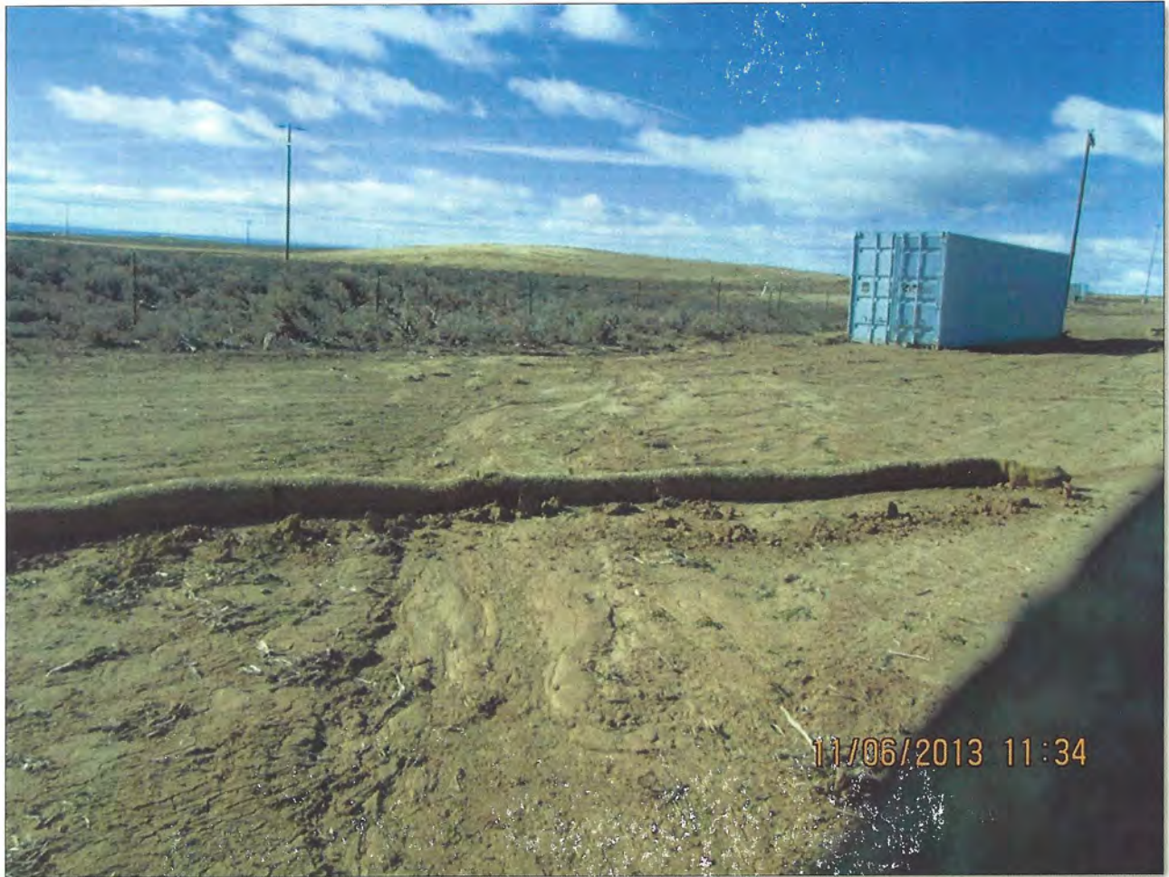
Photo Number 22: This a view looking down gradient (south) where the diversion ditch that goes around the east side of the site's ponds enters native ground. This area was recently reclaimed (seeded) earlier this fall (2013) and was tested by the numerous precipitation events that occurred in September and October. While evidence of the run off associated with those precipitation events is evident in this picture, the reclamation held-up extremely well. Once vegetation is established here, this area will most likely be well-equipped to absorb any/all storm events that may occur.
