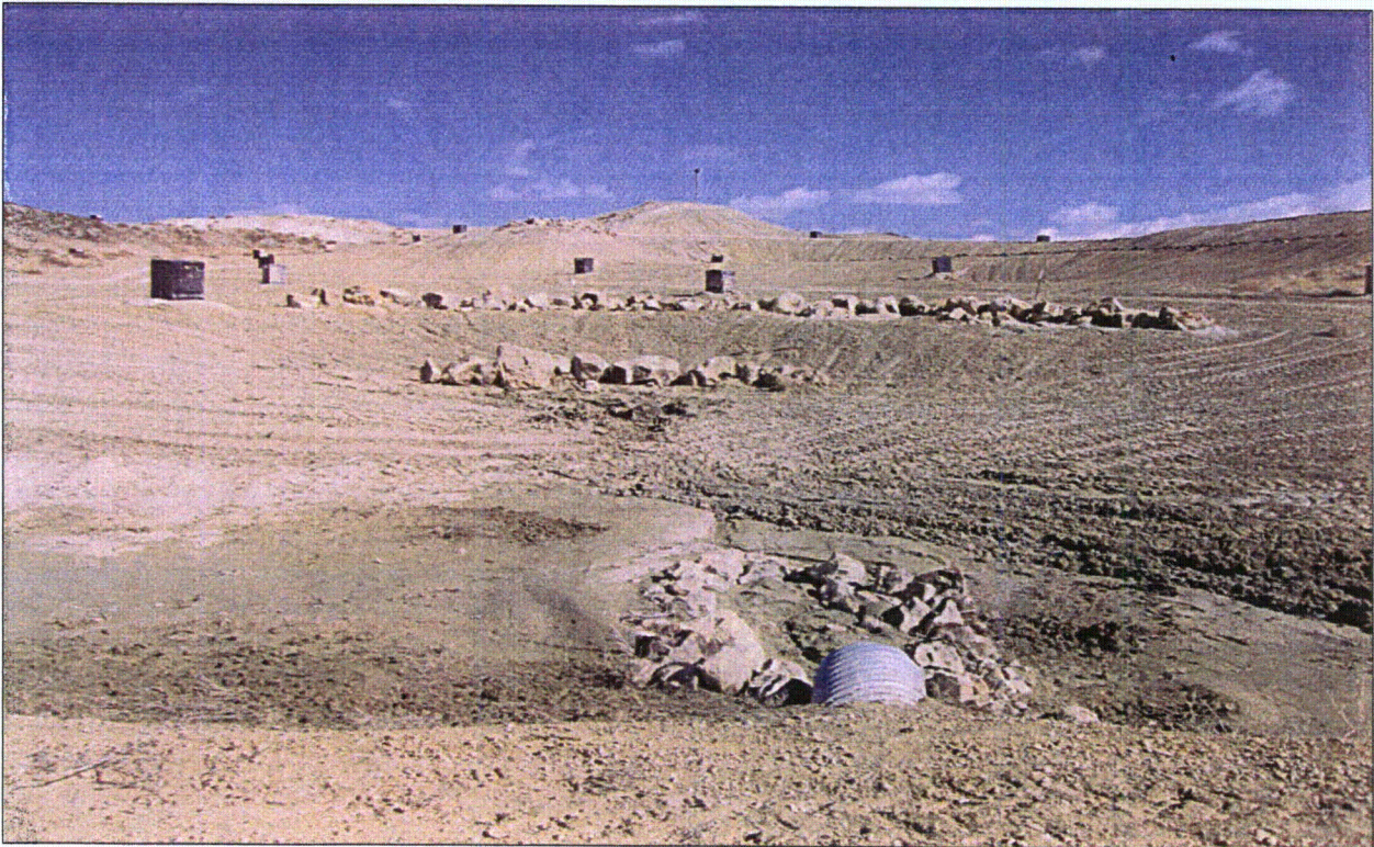
Photo #6 – View rock energy dissipater type structures in CR Mine Unit 8-4/5.
