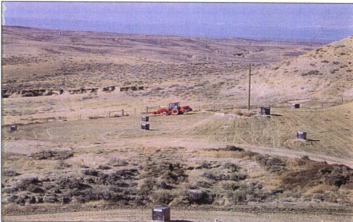
Photo #4 – View of interim seeding operations in CR Mine Unit 8-4/5.
