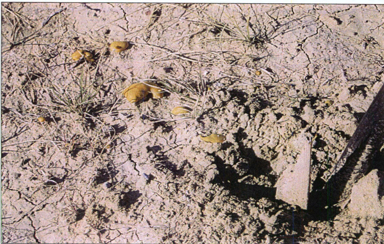
Photo #11 – View of remnant Styrofoam sealant next to temporarily surface capped pilot hole.
