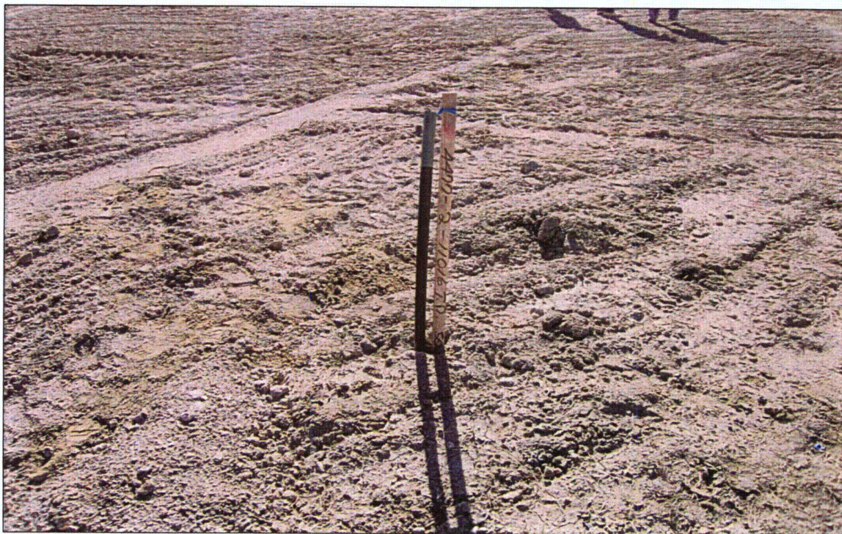
Photo #10 – Temporarily surface capped pilot hole marking in CR Mine Unit 10B.
