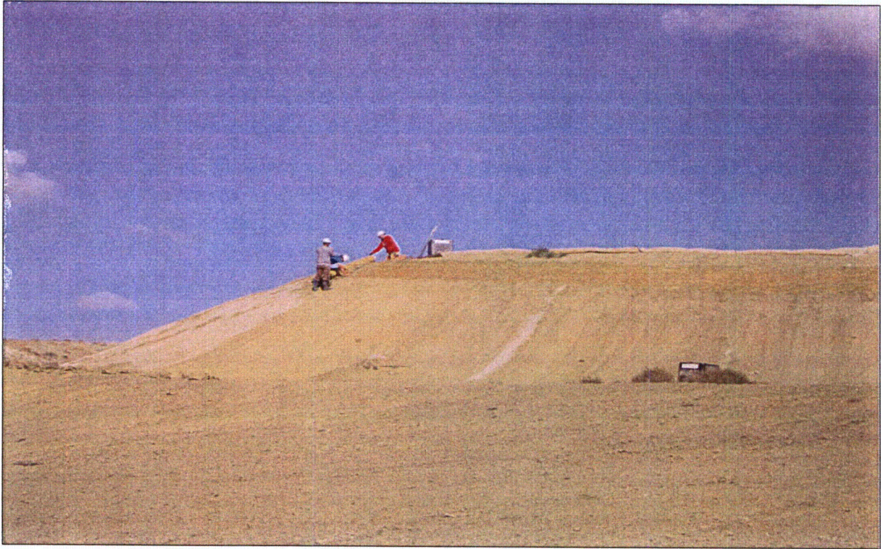
Photo #5 – Placement of erosion control matting in CR Mine Unit 8-4/5.
