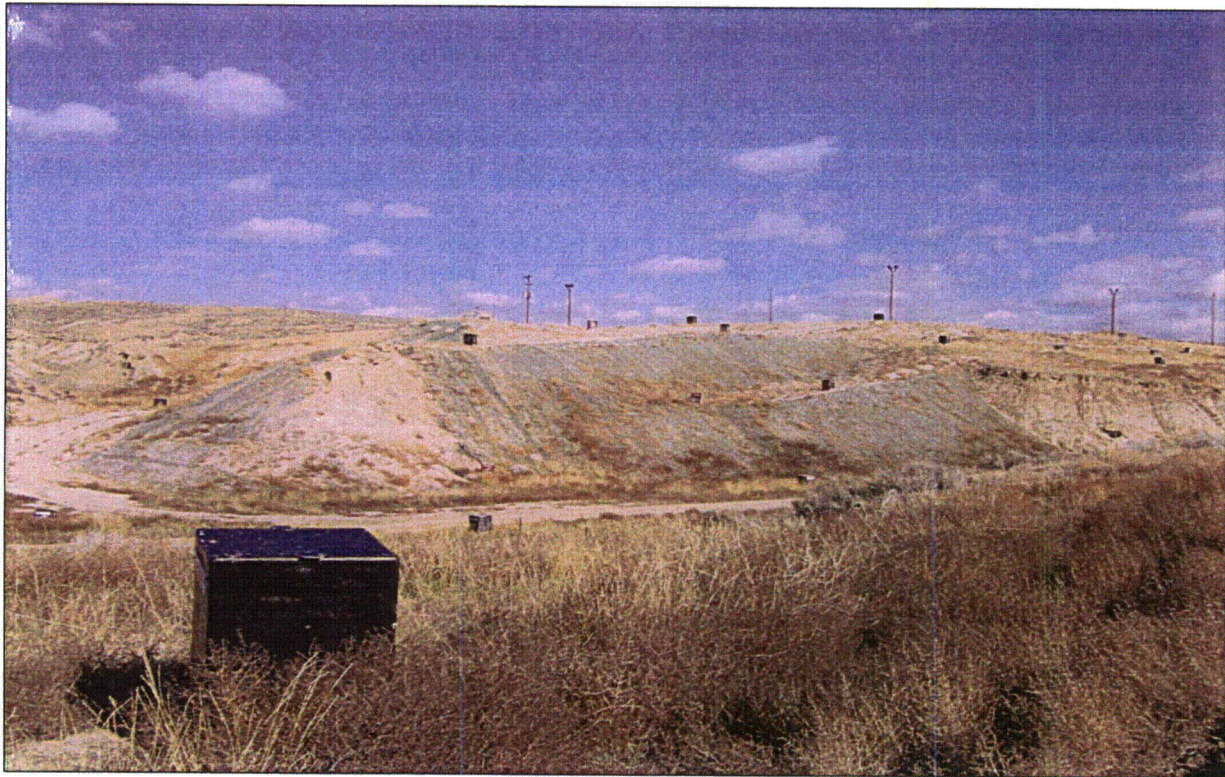
Photo #3 – View of slope erosion control utilizing matting in CR Mine Unit 8.
