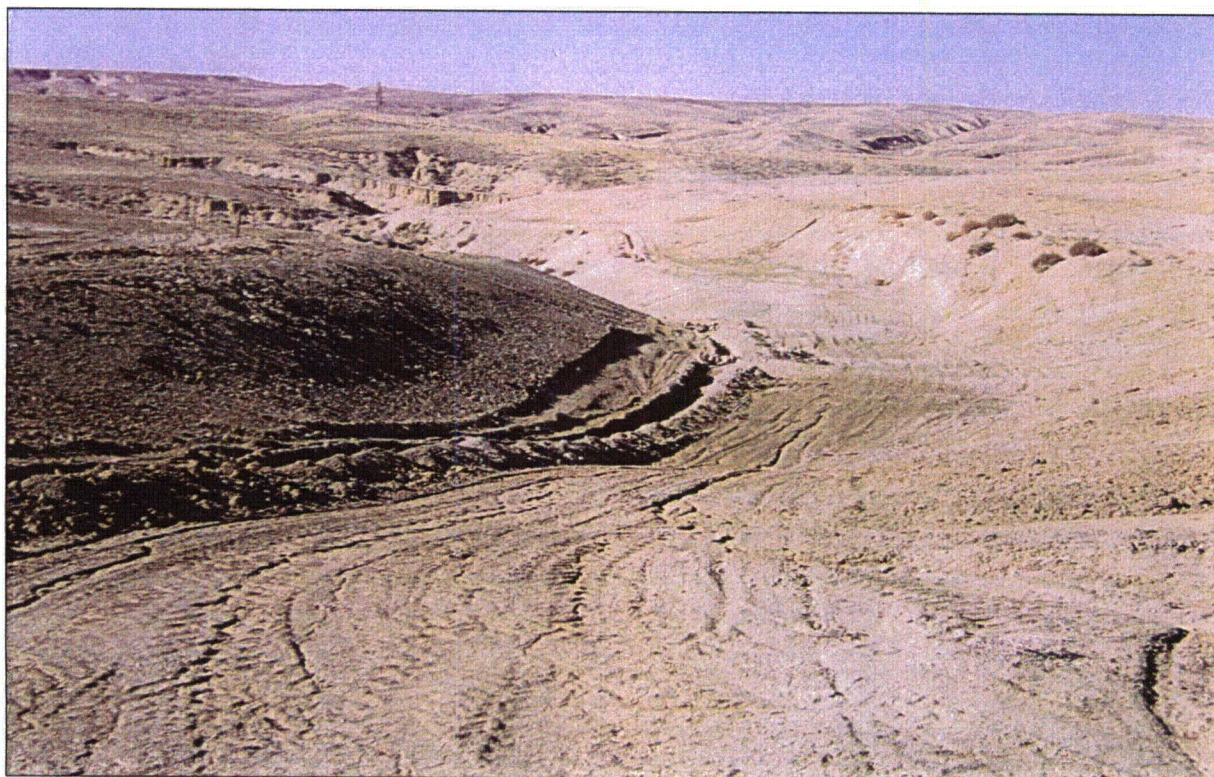
Photo #12 – Disturbance requiring additional sediment control in CR Mine Unit 10B.
