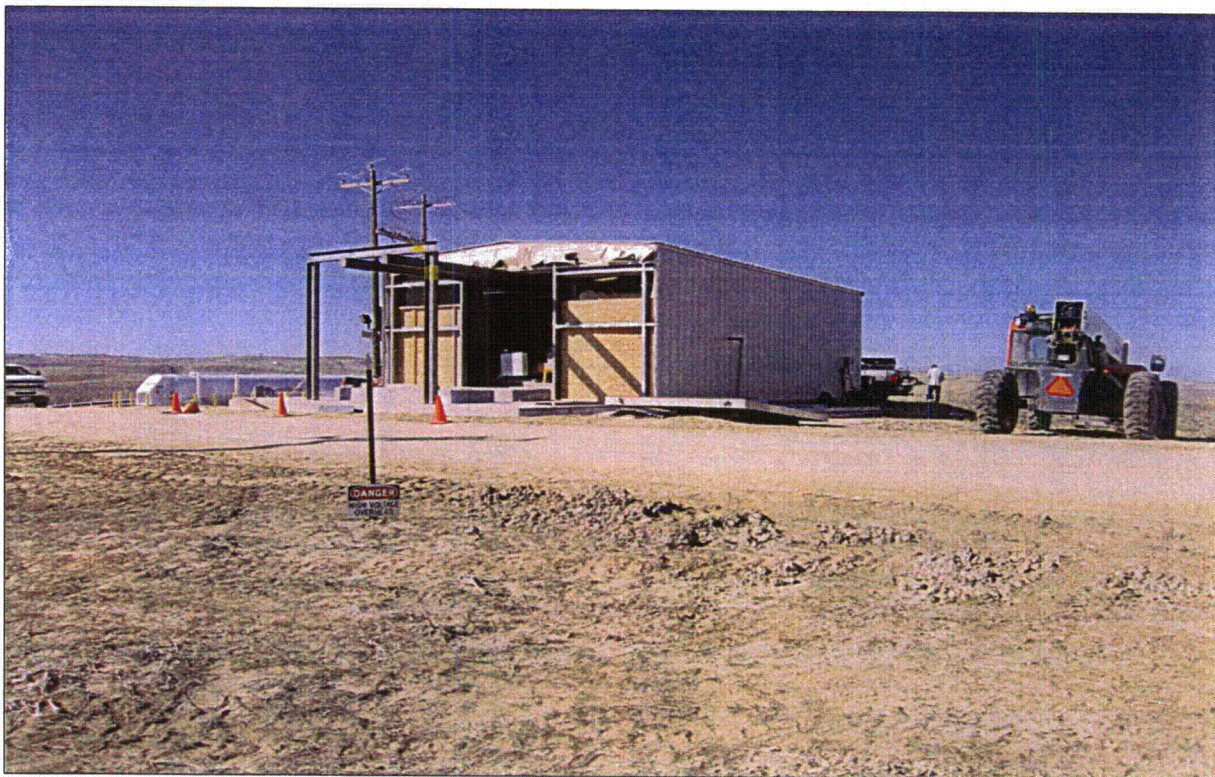
Photo #2 – Construction of addition onto CR Mine Unit 8 Booster Station.
