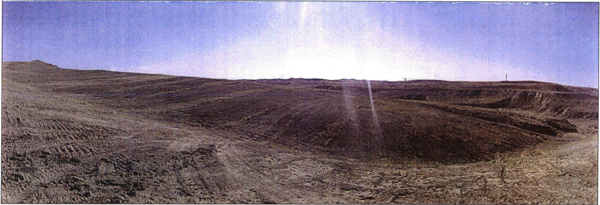
Photo #14 – View looking southwest of wellfield pipeline removal area Irigaray Mine Unit 9. Radiation survey point markers are present along the former pipeline corridors but not visible in this photograph.
