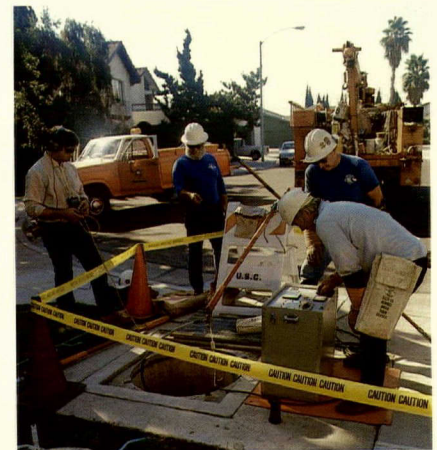
Apprentice Line Mechanic Mitch Schroeder and Cable Splicers Barney Allen, Bob Durbin and Bob Holden use fault locator equipment to detect underground electric cable faults.
