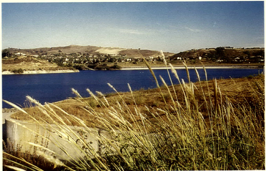
Colorado River water traverses the desert via MWD's aqueduct and is stored in Anaheim's 920 million gallon Walnut Canyon Reservoir prior to treatment.
