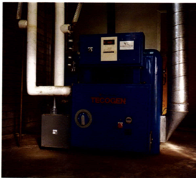
In 1989, the company began to purchase and operate cogeneration units for commercial customers.
