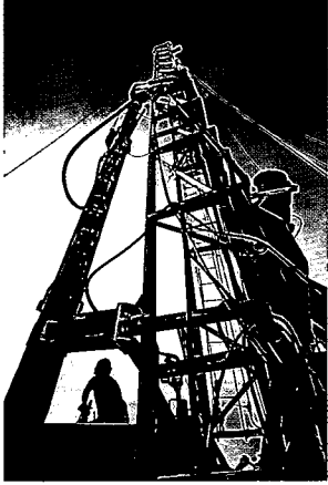
On Center Street, Riverside Public Utilities drills a new domestic water well. Over 90% of the city's water supply comes from wells which are publicly owned through Riverside Public Utilities.
