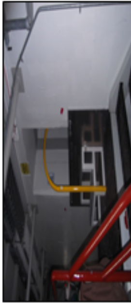
Brunswick Control Building Door
