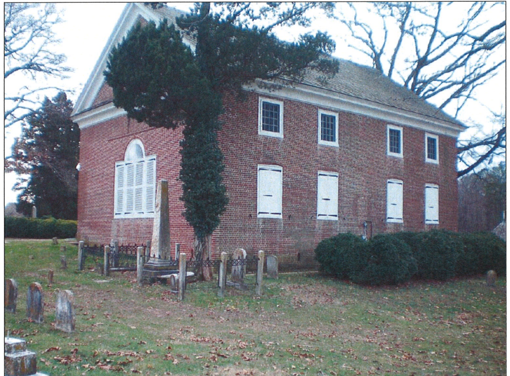
Resource 64: Old St. Anne's Church, 15 East Green Street, Middletown State/National Register Listed Visibility: The cooling tower is visible from this location
