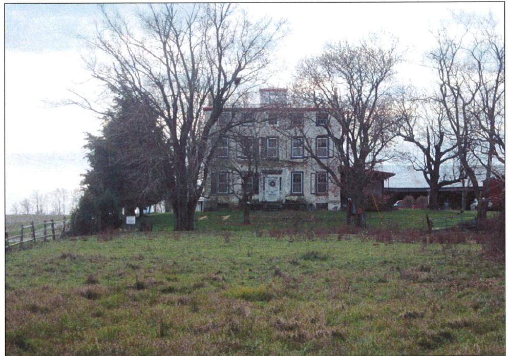
The residence at 349 Fort Elfsborg Road is located at the edge of the 4.9-mile study area for the architectural resources reconnaissance-level field survey. The two-and-a-half-story masonry residence has a hipped roof and is surmounted by a cupola. It exhibits elements of both the Greek Revival and Italianate styles, and likely dates to the mid 19th century. The windows throughout the house contain six-over-six-light double-hung sash with the exception of the eyebrow windows at the top story level. The proposed cooling tower location appears to be visible from the potential resource.
