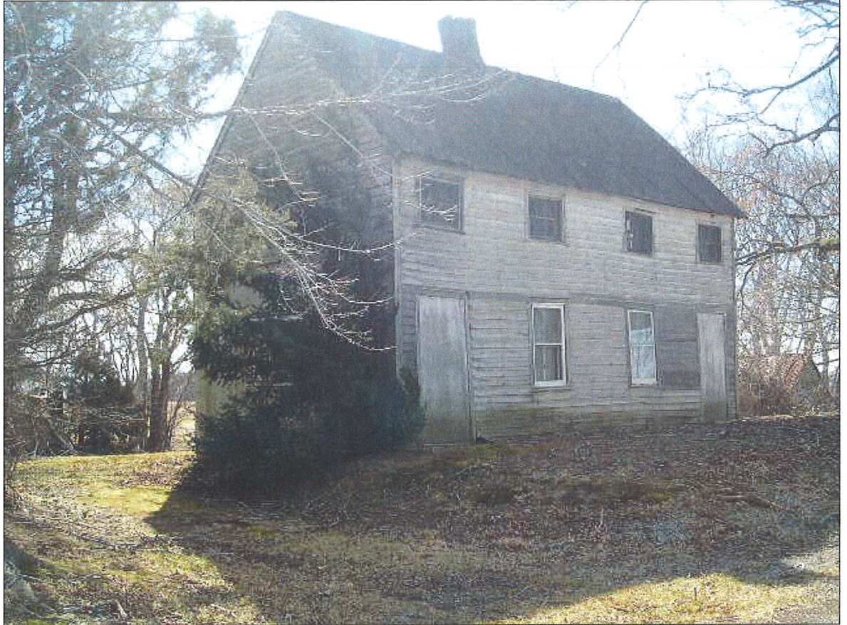
This two-story wood-frame vernacular house is located at 50 Cedar Swamp Road in Townsend, Delaware. Likely constructed in the early 19th century, the house has a central brick chimney and a steeply pitched roof. It is clad in wood clapboards. Entries are located at either end of the front façade. The ground-story windows appear to have been replaced in the late 19th century with two-over-two-light double-hung sash. The smaller upper-story windows retain three-over-three-light sash. The house appears on the 1868 Pomeroy & Beers Delaware State Atlas as belonging to W.S. Deakyne. The proposed cooling tower location appears to be visible from the potential resource.
