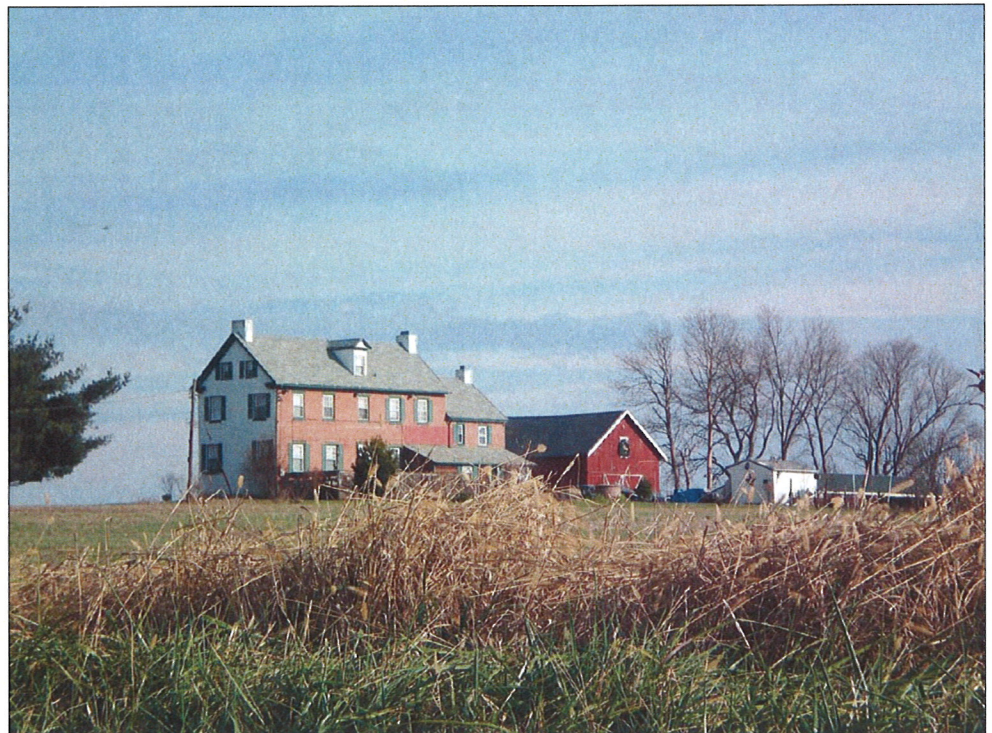
Resource 17: Idalia Manor – US Route 13, Mount Pleasant State/National Register Listed Visibility: The cooling tower is visible from this location.
