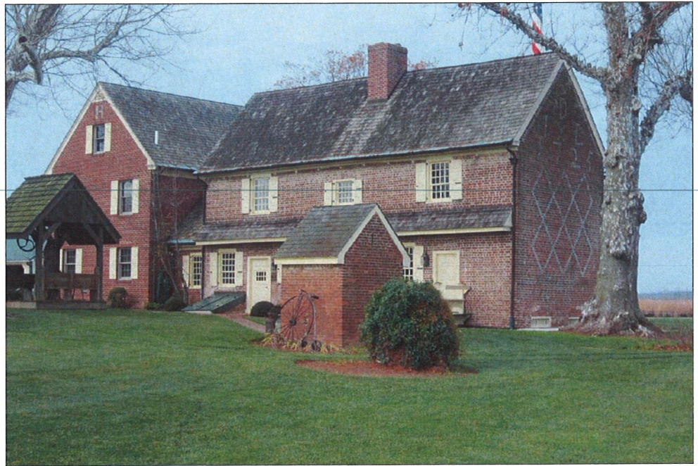
The John Maddox Denn House, located at 112 Poplar Street in Lower Alloways Creek Township, Salem County, New Jersey. Constructed in 1725, this patterned brick house features the construction date of 1725, Denn's initials, and a diamond pattern in glazed brick in the gable end. The interior is an open floor plan with a central fire place. The portion of the structure to the left is a mid- to late-20th century addition. The Denn House was surveyed by the Historic American Building Survey (HABS) in 1933. According to MACTEC's visual assessment, the proposed cooling tower is not visible from the resource.
