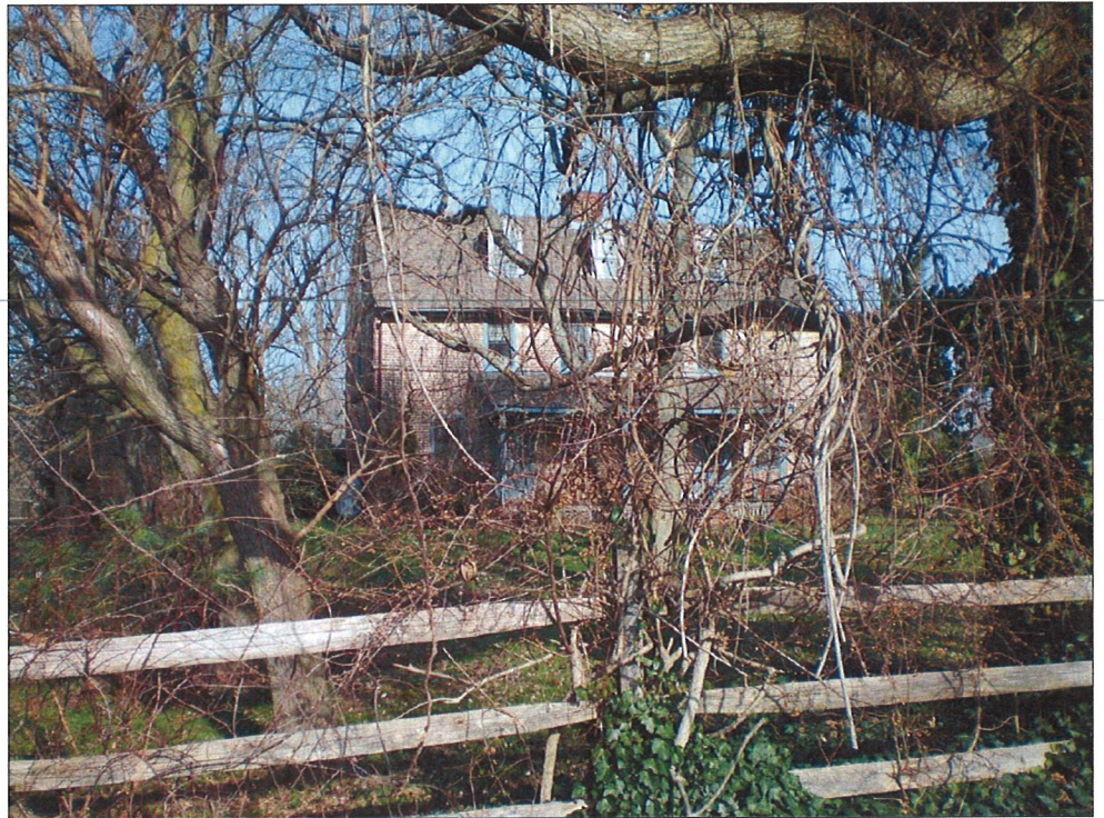
Resource 25: Robert Grose House – 1000 Port Penn Road, Port Penn State/National Register Listed Visibility: The cooling tower is visible from this location
