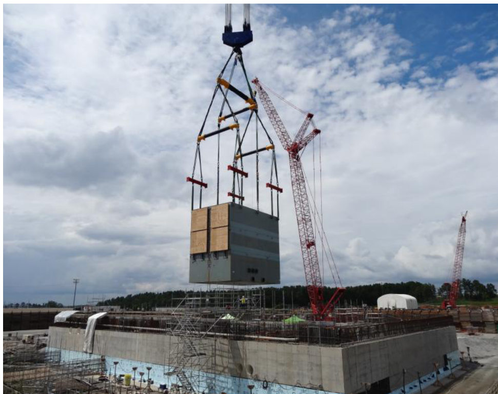
Condenser B Lower Shell July 2013 700 Tons
