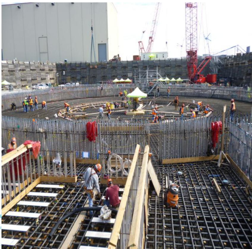
Shield Building Rebar, looking North to South
