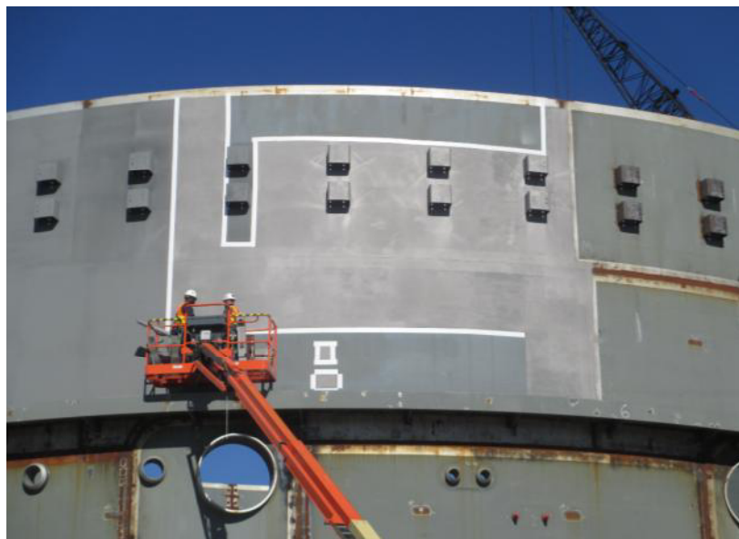
Steel surface preparation for inorganic zinc application
