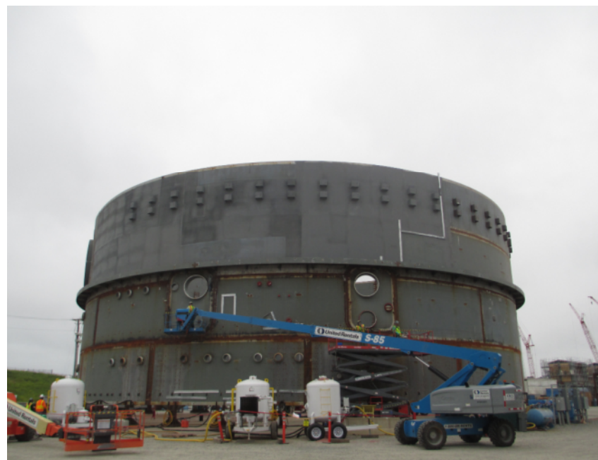
Inorganic zinc application in progress on U2 CV Ring 1
