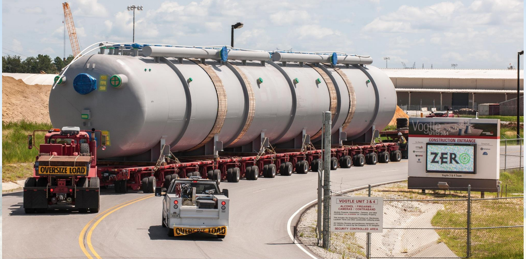
Plant Vogtle Unit 4 deaerator arriving to construction site
