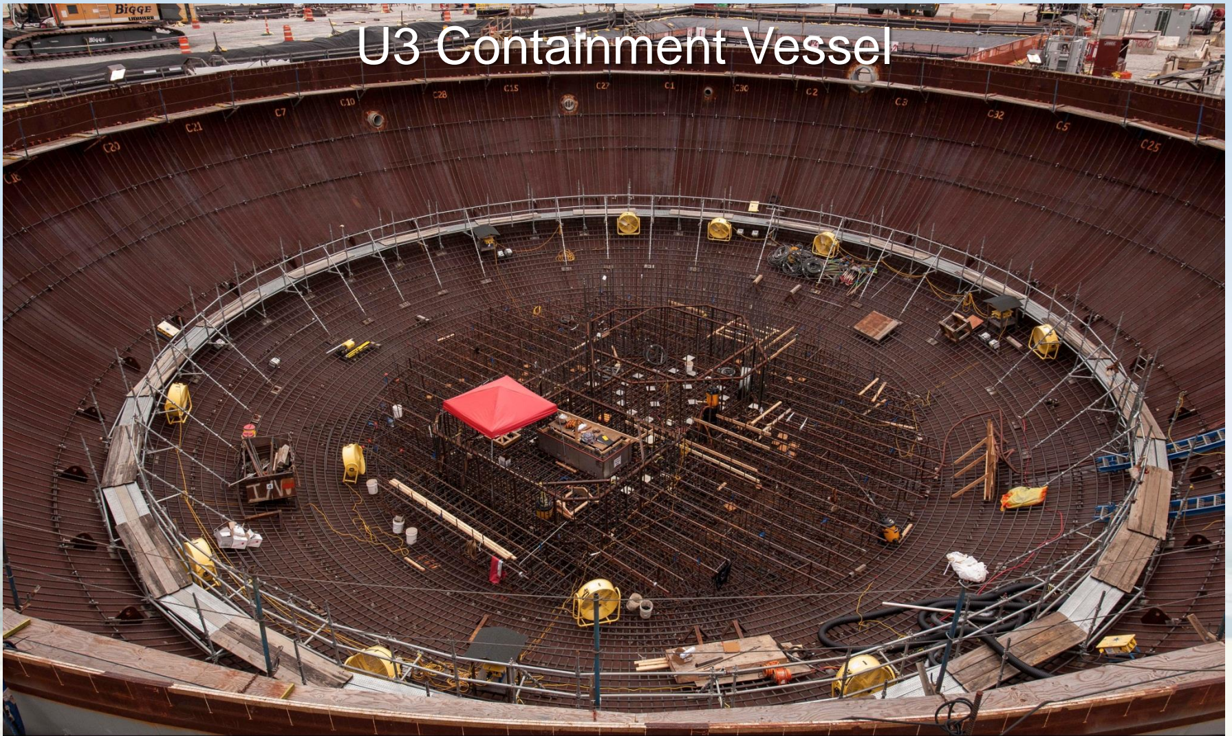
Plant Vogtle Unit 3 containment vessel bottom head, located inside nuclear island
