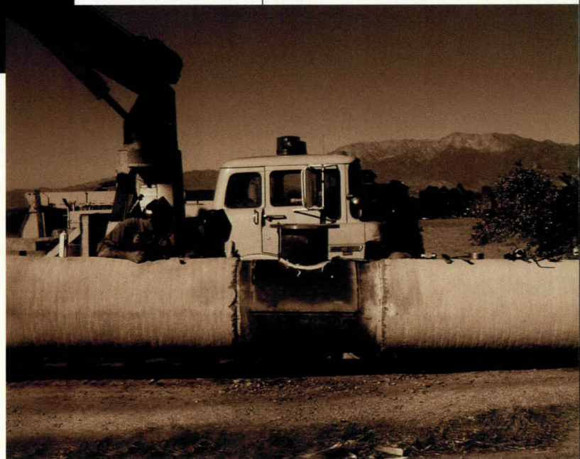
Dufferin Avenue water transmission line construction.
