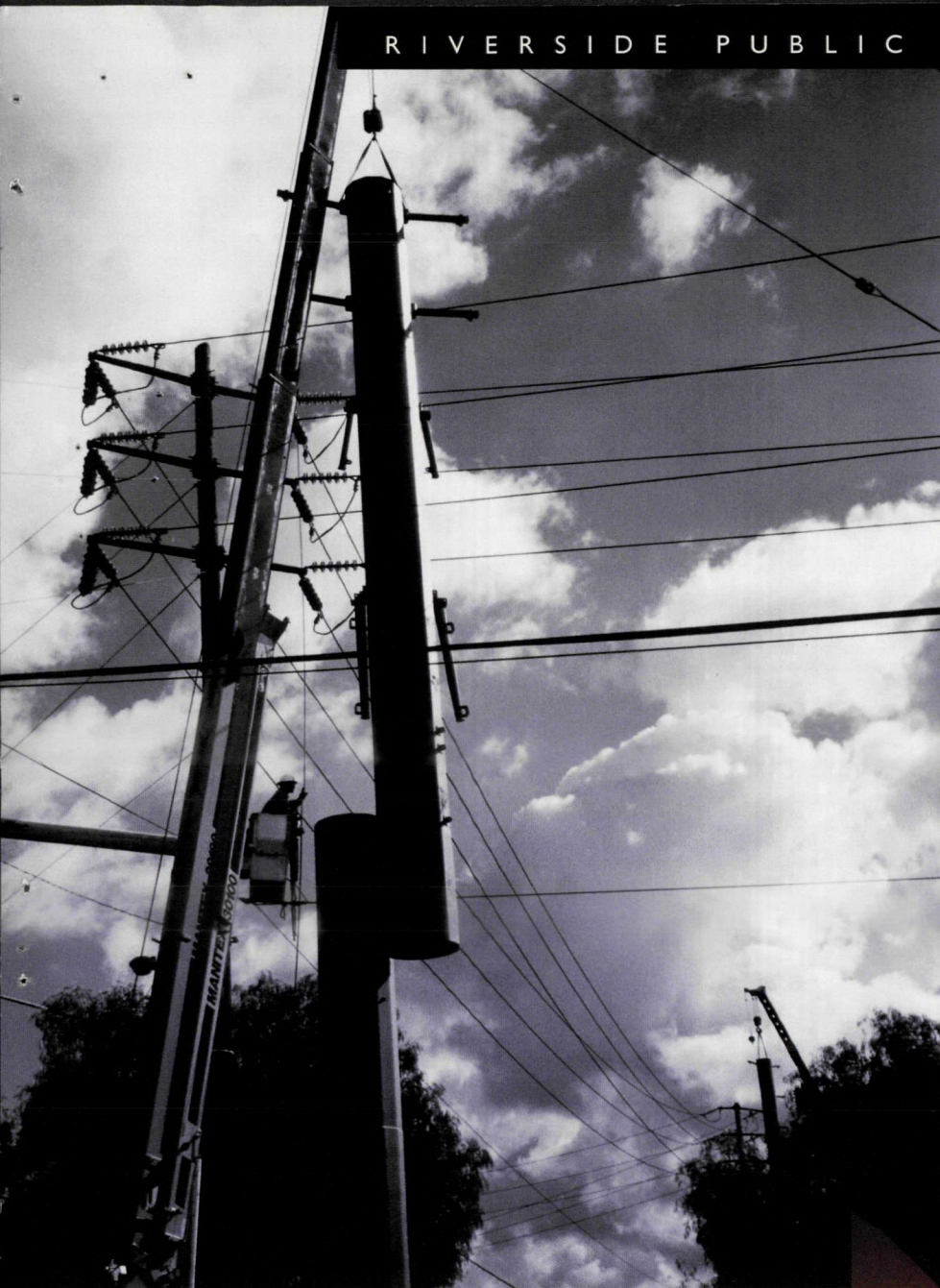
Construction of Vista-Freeman 69kv electric transmission line.
