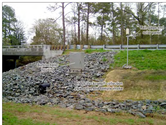
Figure 2. Discharge pipe sampling configuration at the Black River site.
