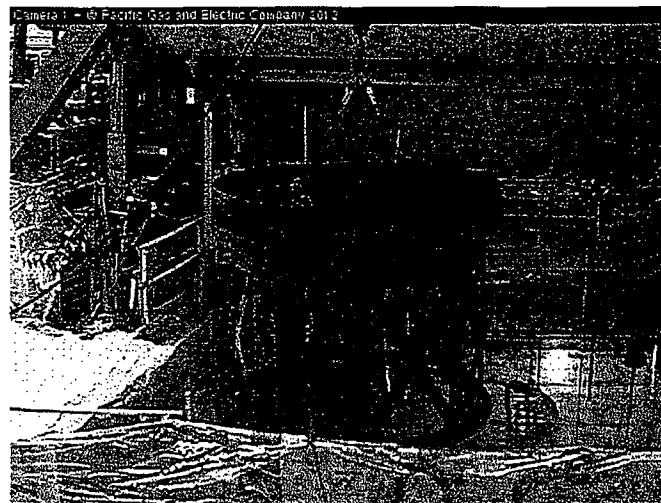
Lower core shroud removed March 2013
