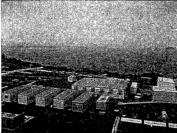
Installation of planning trailers 2008
