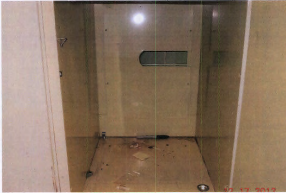
Health Physics Laboratory (Room 1264) - Radioactive Material Storage Cabinet (Room 1264) Post - Closeout
