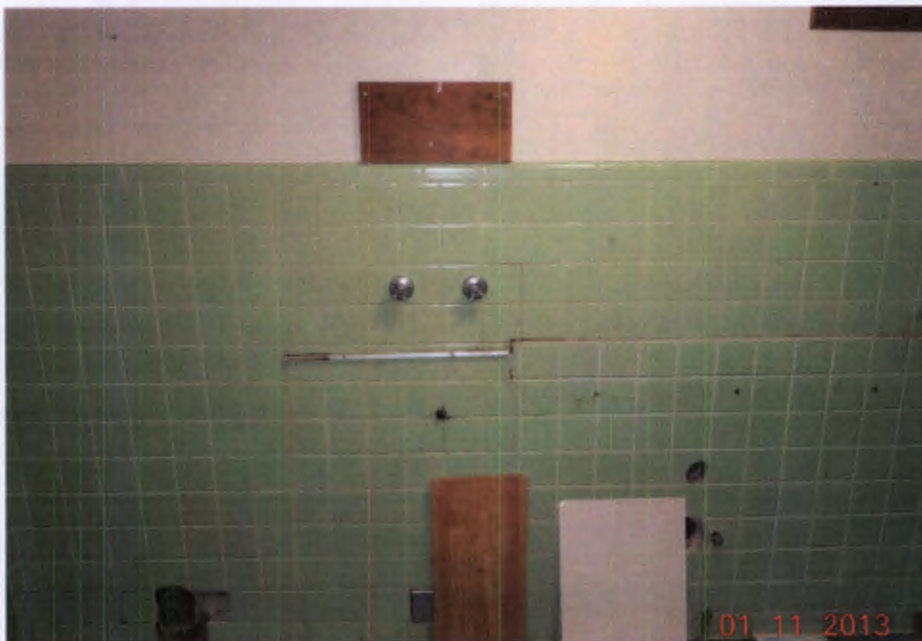
Health Physics Radioactive Material Storage Room (Room 1265A) Post - Closeout
