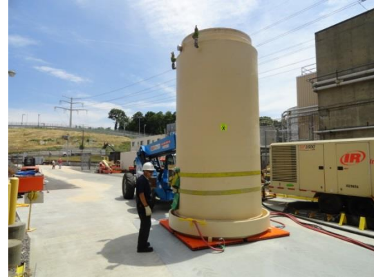
HI-TRAC with loaded STC moved out of U3 on air pads
