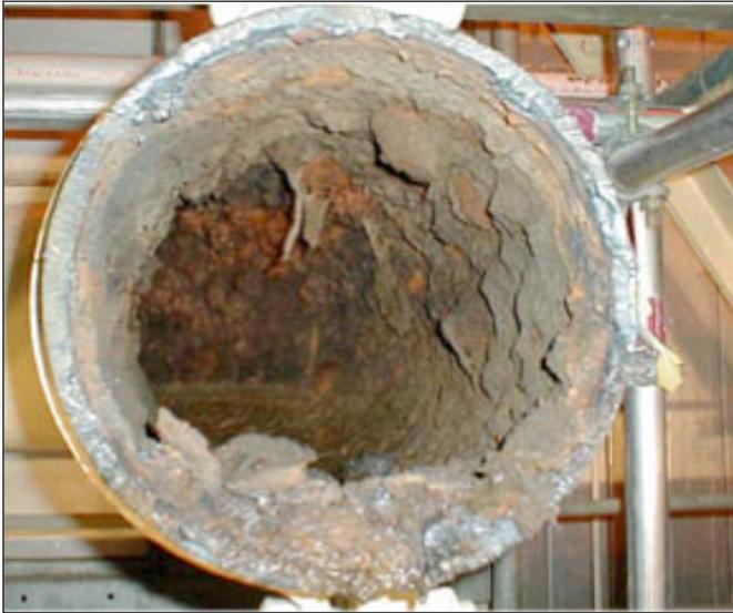
Figure 9.23 Corrosion and biofouling of carbon steel service water system piping
