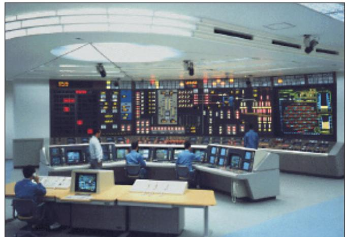
Figure 10.1 Highly integrated control room
