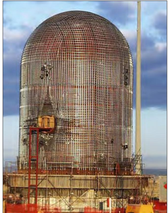
**Figure 8.9 Prestressed concrete containment vessel model tendon sheaths at Sandia National Laboratories**
