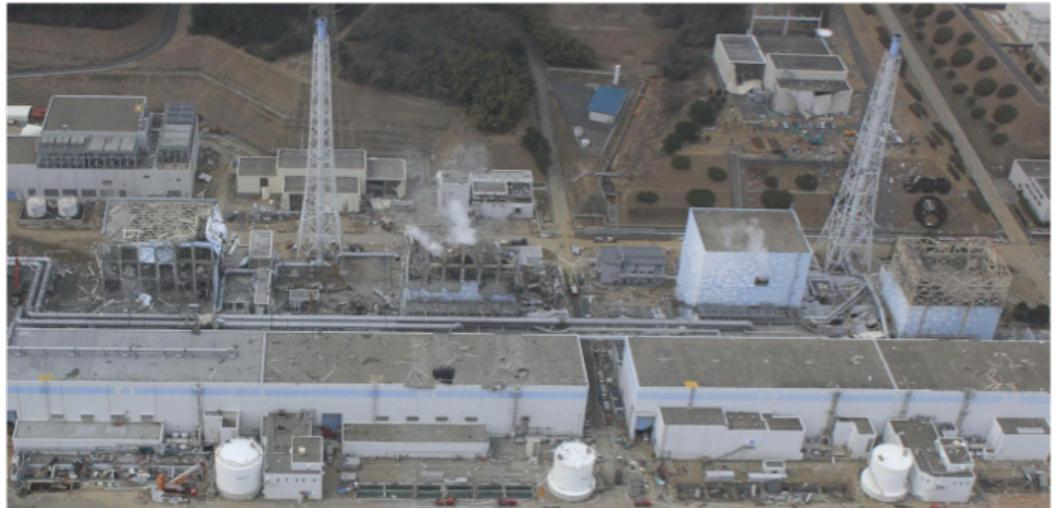
**Fukushima Units 1, 2, 3, and 4 after the accident showing extensive damage to the reactor buildings**
