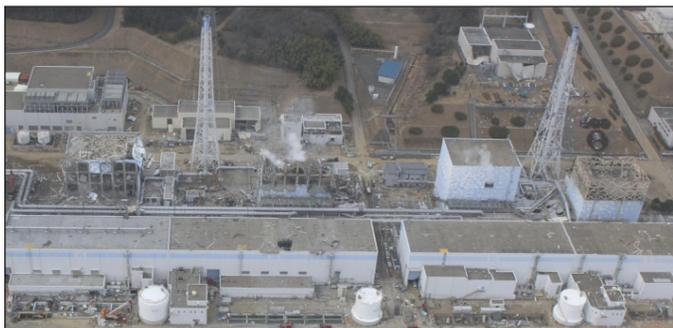
Figure 11.7 Fukushima Units 1, 2, 3, and 4 after the accident showing extensive damage to the reactor buildings
