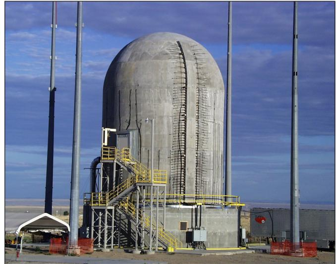
Figure 12.14 Completed pre-stressed concrete containment vessel 1:4 scale model at SNL (Source: Figure 52, NUREG/CR-6906 (SAND2006-2274P))
