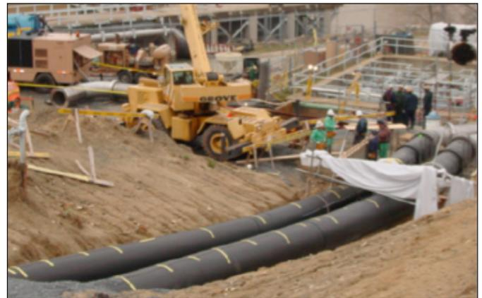
Figure 9.24 Installation of underground Class 3 safety-related HDPE piping
