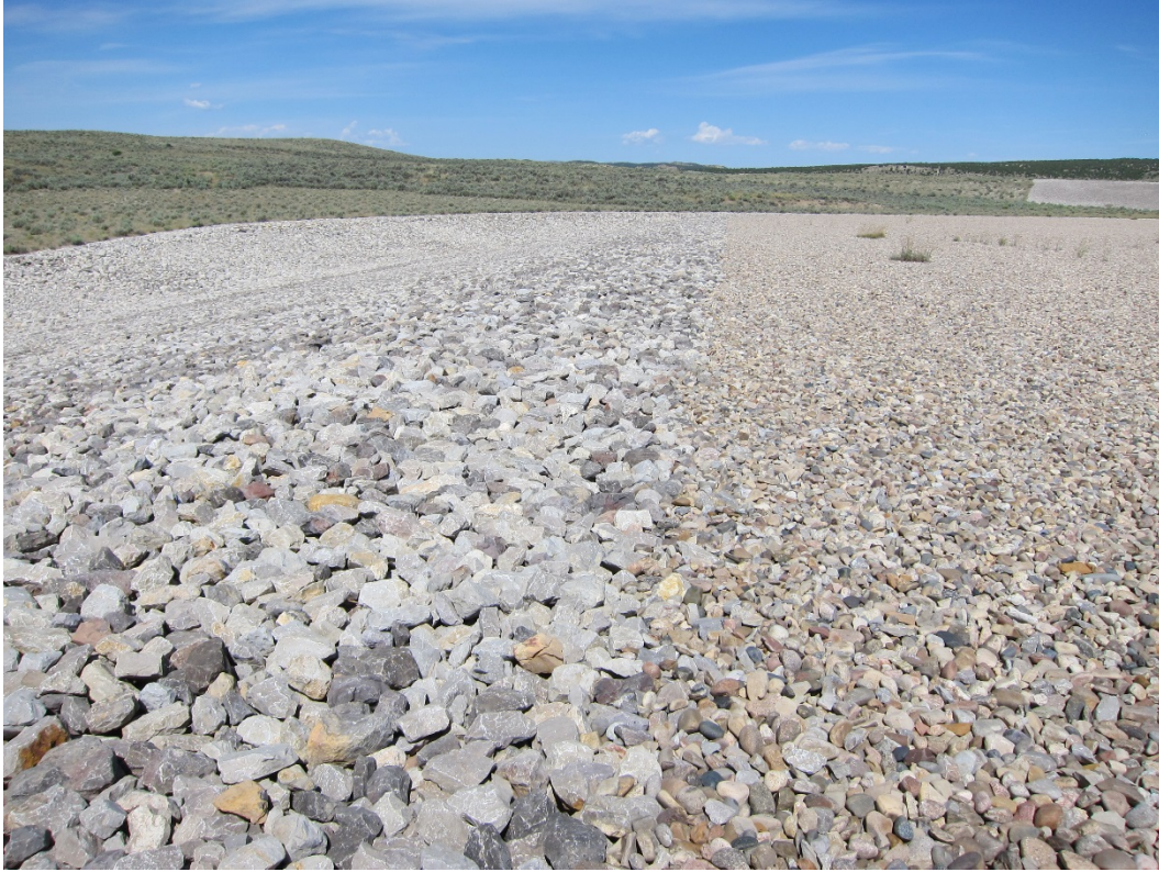
Figure 3: Diversion channel (left) and top of cell (right); southwest side of cell
