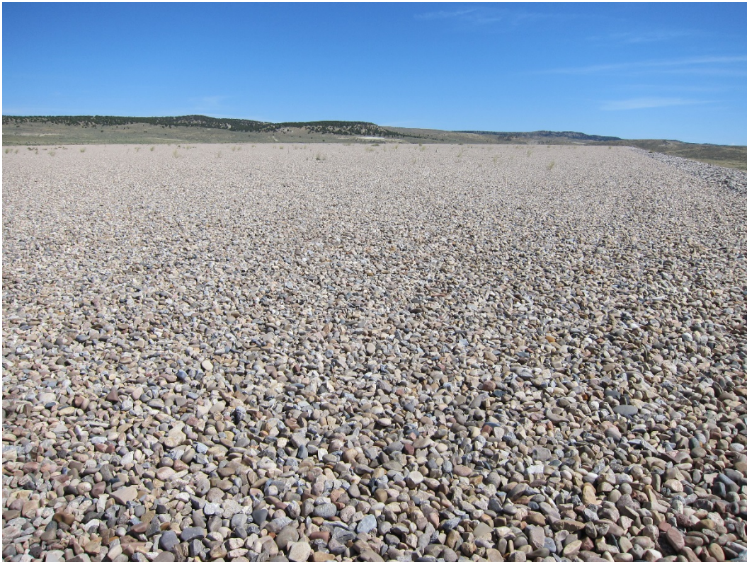
Figure 2: Top of Maybell disposal cell (looking north)
