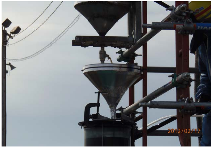
Figure 6 –Grout Addition Funnel
