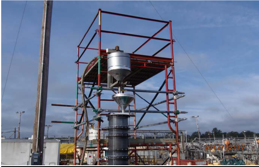
Figure 5 – Top of Mock-up Model and Grout Addition Funnel
