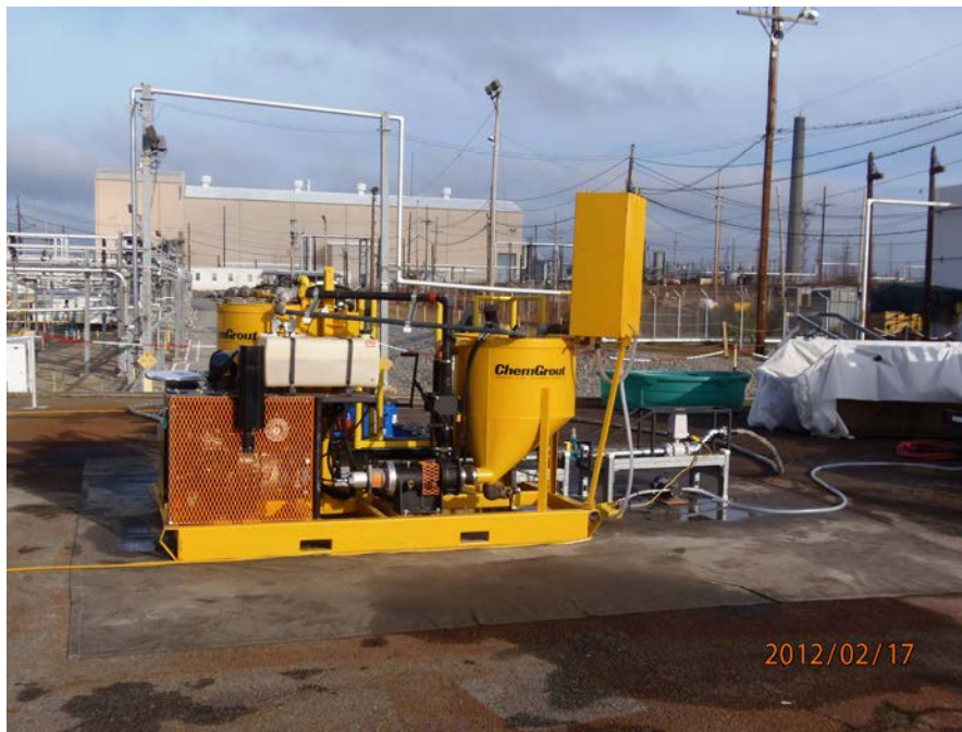
Figure 2 – Test Equipment For Grout Property Test
