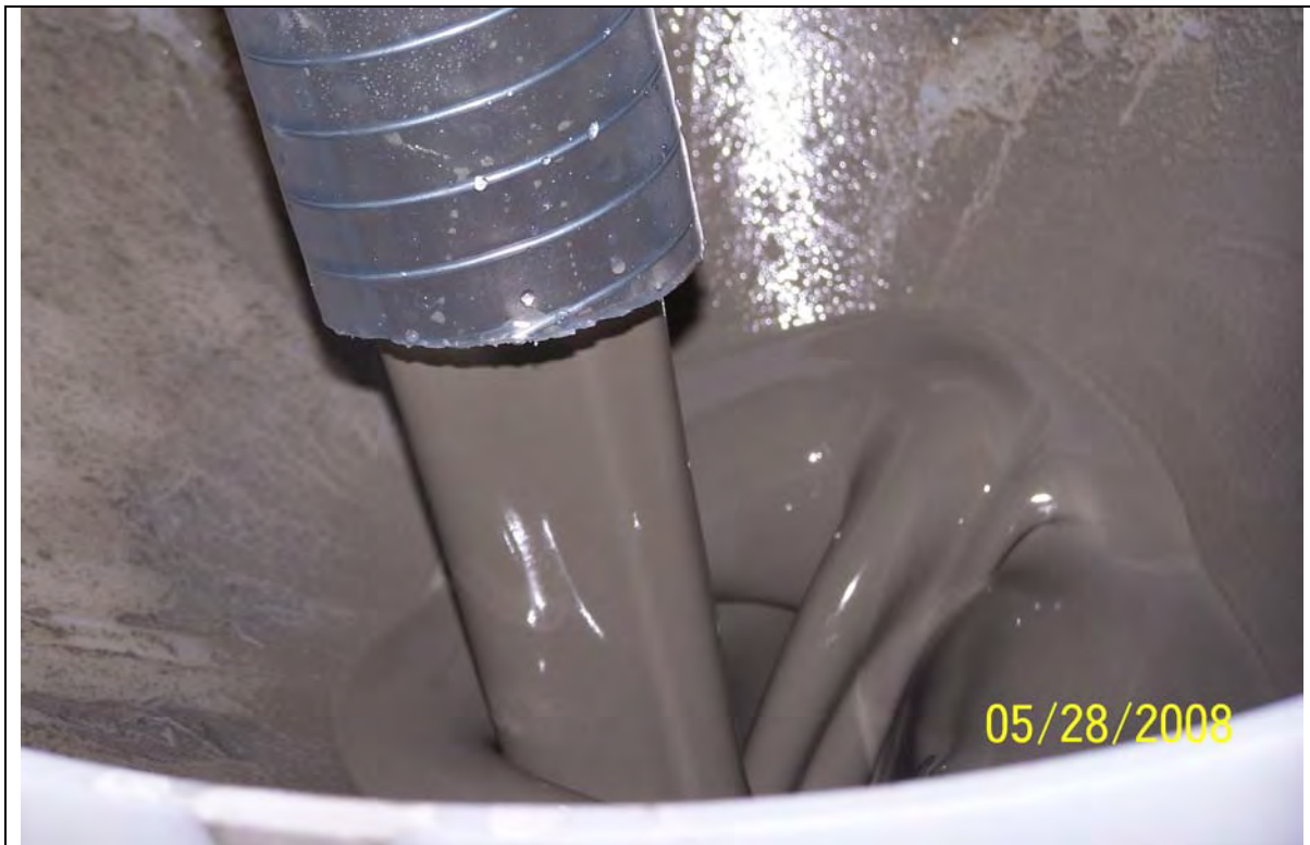
Figure 3-14 Typical Grout Discharging the Horizontal Cooling Coil Assembly
