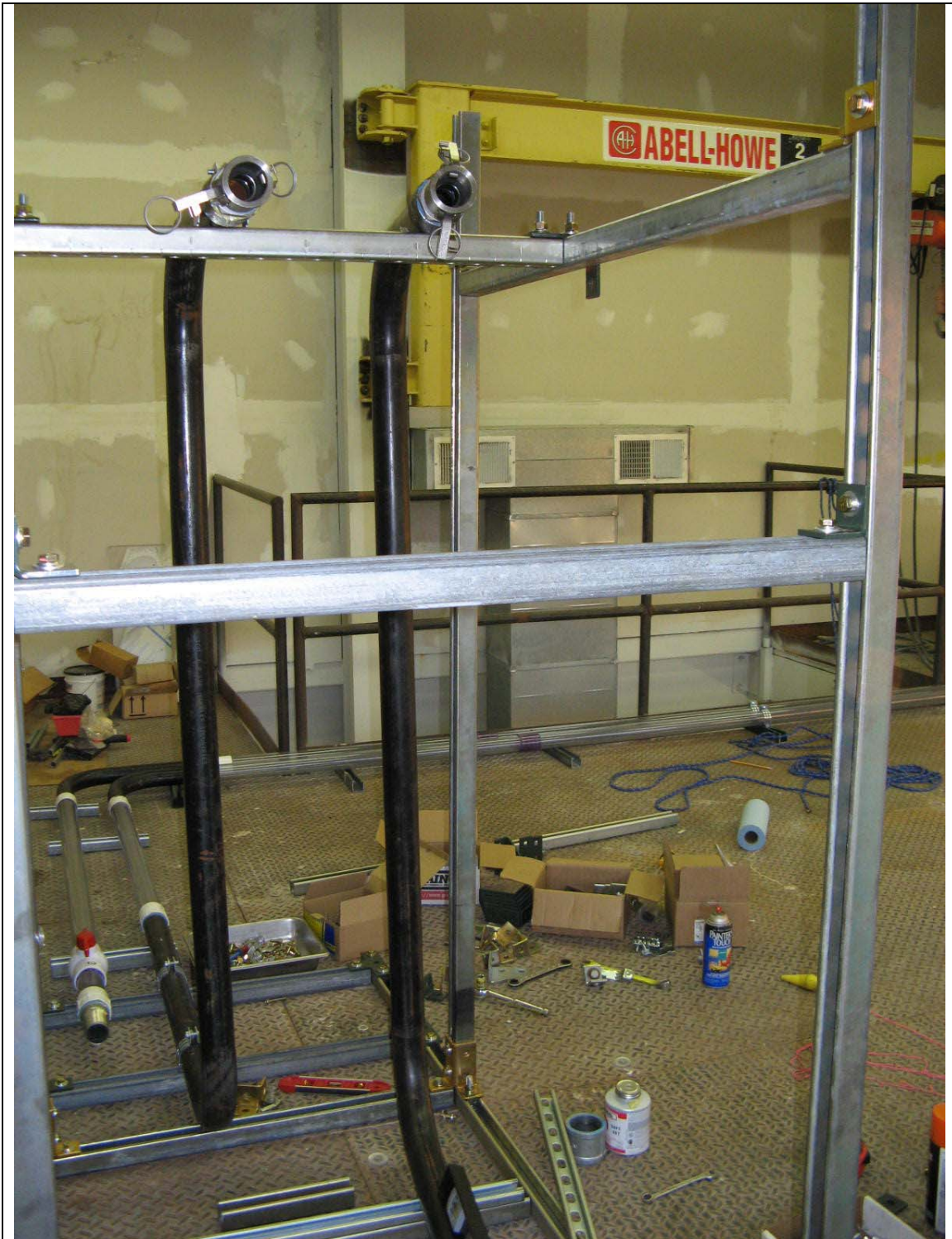
Figure 2-9 Vertical/Horizontal Cooling Coil Assembly - Third Floor
