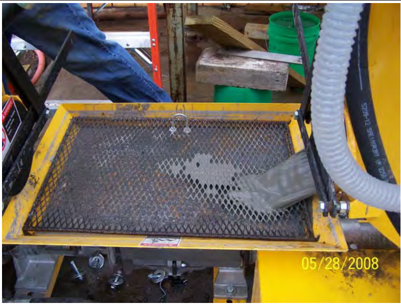
Discharge of grout over pump section hopper grating
