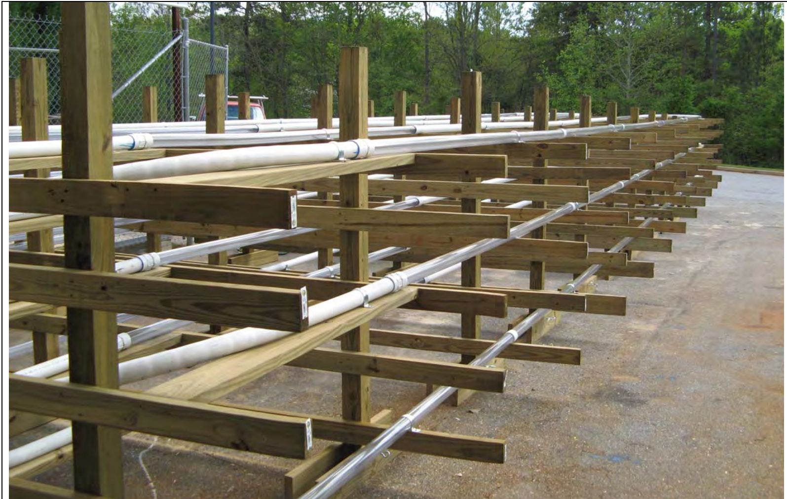
Figure 2-10 Horizontal Cooling Coil Assembly – Outside – Side View
