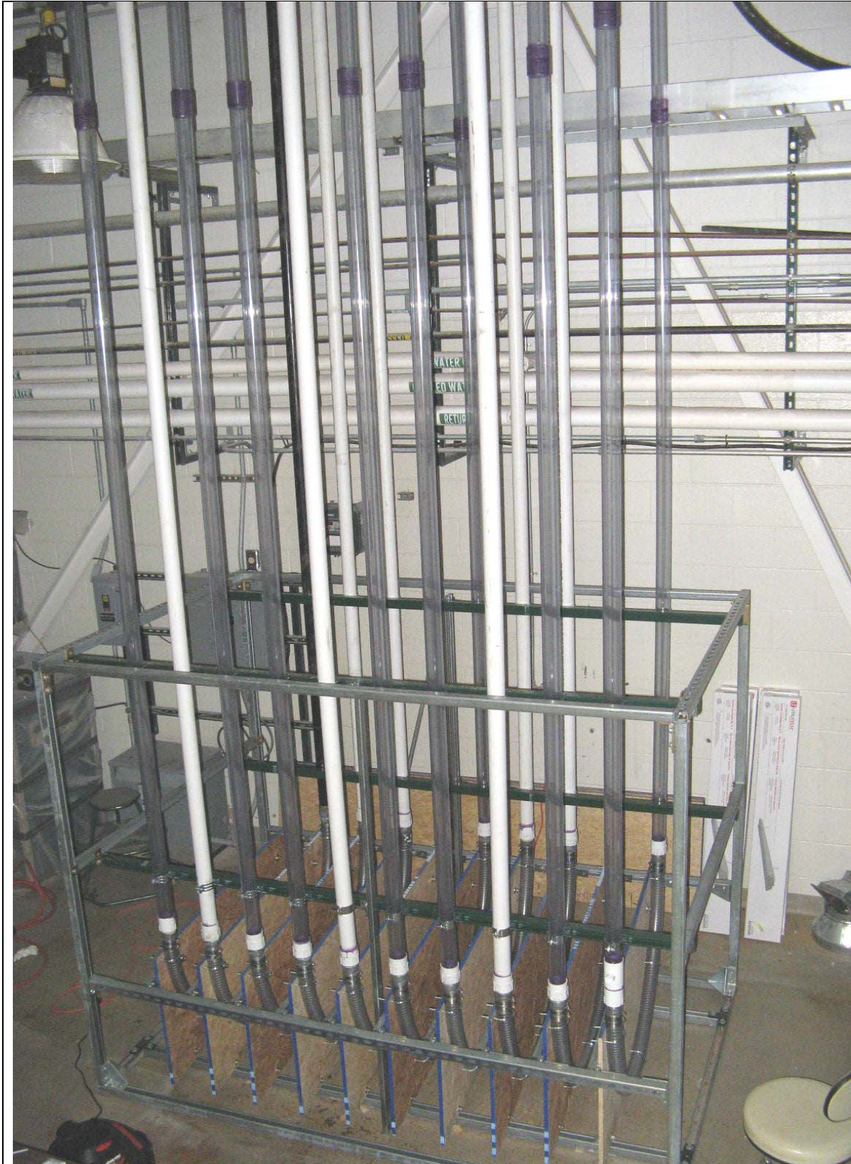
Figure 2-7 Vertical Cooling Coil Assembly - First Floor
