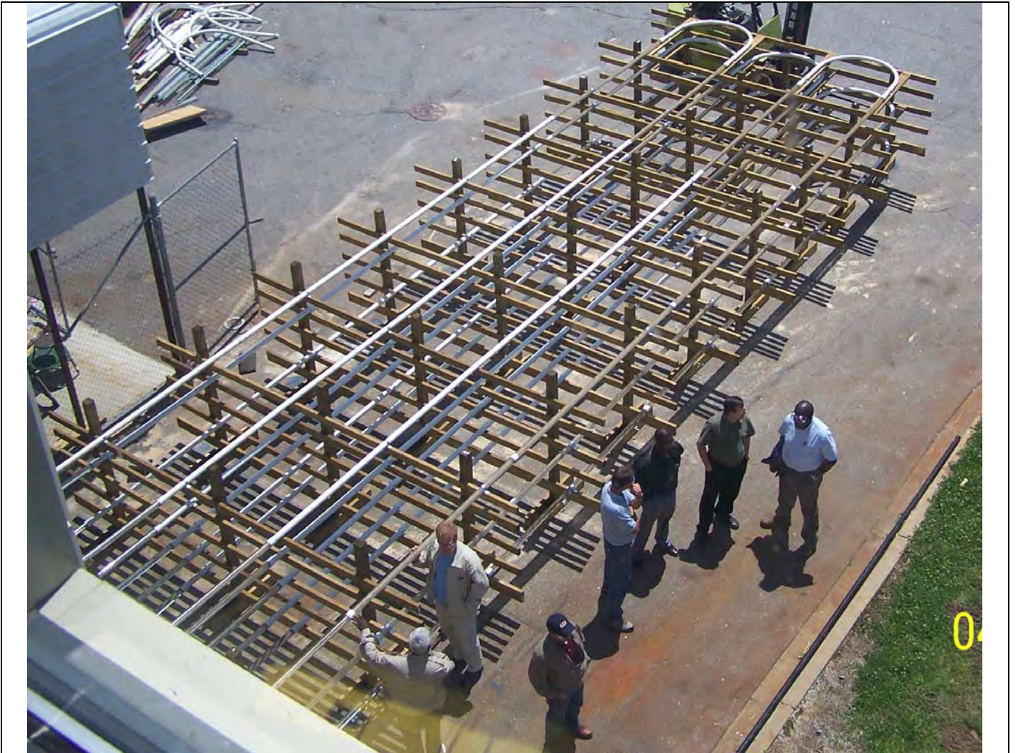
Figure 2-11 Horizontal Cooling Coil Assembly – Outside – Top View
