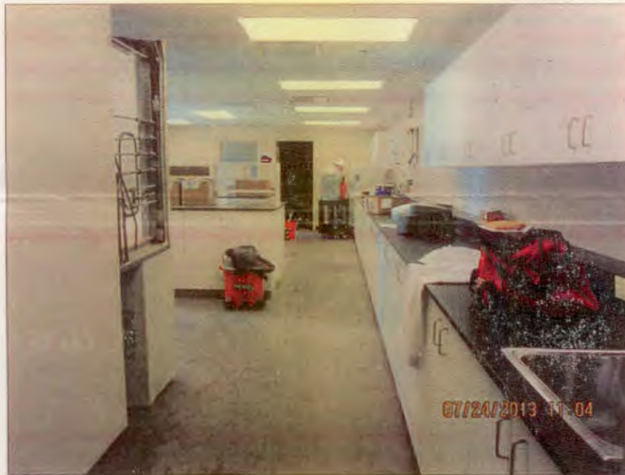
Photo Number 3: This depicts the lab in the Plant Building.
