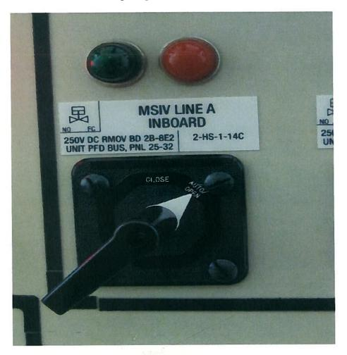
If the TRANSFER SWITCH, 2-XS-1-14, is placed in EMERG with 2-HS-1-14C handswitch on panel 2-25-32 positioned as shown above, the A INBOARD MAIN STEAM LINE ISOLATION VALVE, 2-FCV-1-14, will \_\_\_\_\_.
