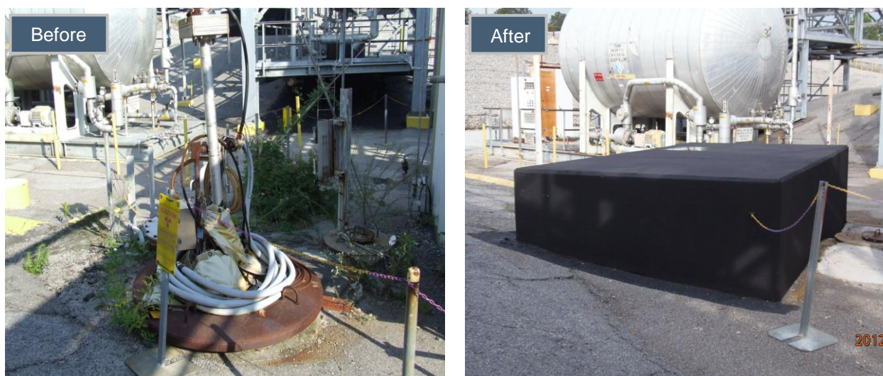
Figure 3.2-2: Typical Riser - Before and After Filling and Capping (Tank 19 Northeast Riser)
