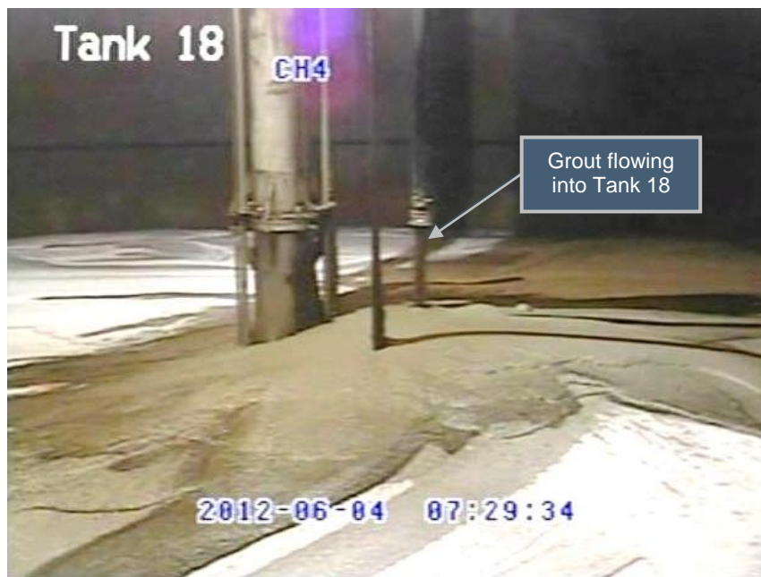
Figure 3.2-1: Bulk Fill Grout in Tank 18 During the Filling Process
