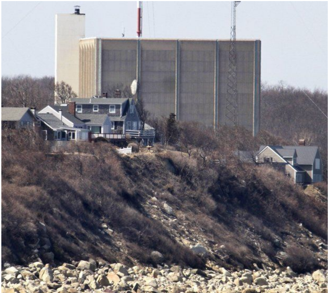
A tower at Pilgrim Nuclear Power Station, in Plymouth, Mass., is seen near the coast of Cape Cod Bay, Wednesday, March 30, 2011. (AP Photo/Steven Senne)
