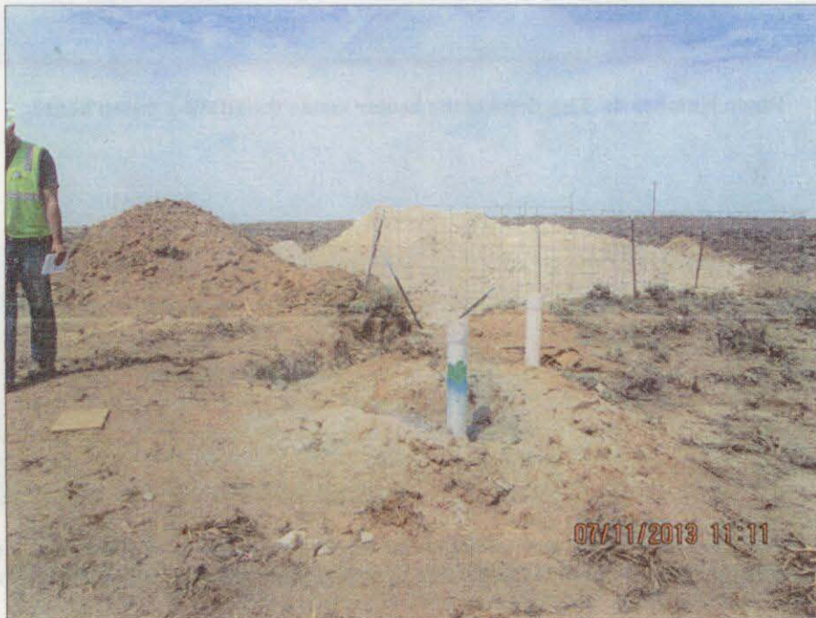
Photo Number 7: This depicts MU2 monitoring ring wells M-206 and M-206a. The associated mud pit is fenced because these wells are outside the MU1/MU2 perimeter fence.
