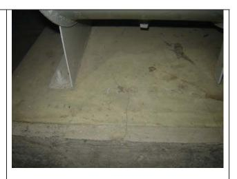
**Note:** Minor hairline cracking in grout pad, away from anchor, OK.
