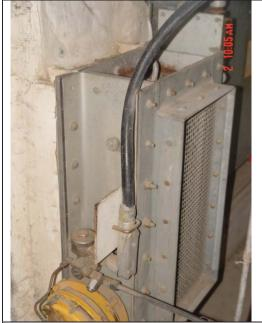
**Note:** AOD anchorage (with missing bolt shown in top left corner)
