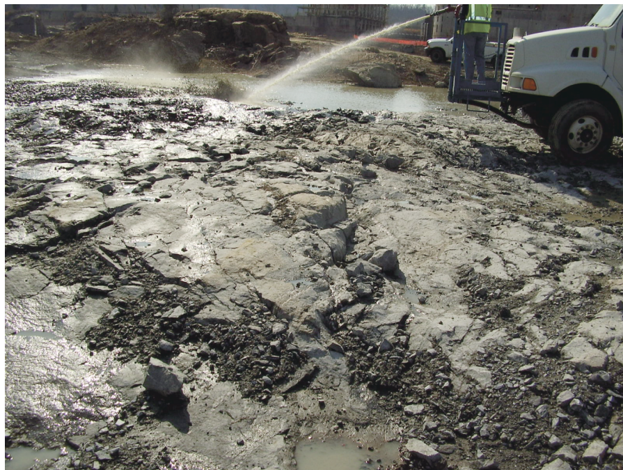
Example of rock cleaning in Unit 2. Water spray is used to remove excessive sediment from exposed rock surface. View towards west, January 3, 2006.
