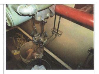
Note: Equipment close to combustibles. (Acceptable for maintenance area under SO-G-91)
