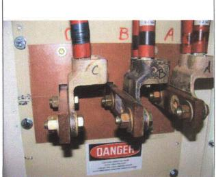
Note: Silver oxide missing on B for panel 1B3A-103.
