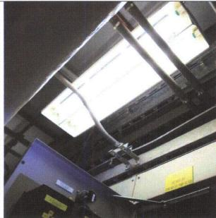
Note: Fluorescent light bulbs posing potential seismic impact hazard.
