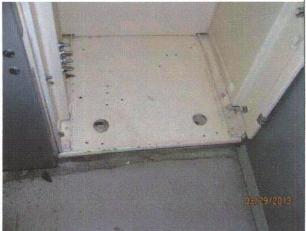
**Note:** Front base of empty cubicle showing plug welds.
