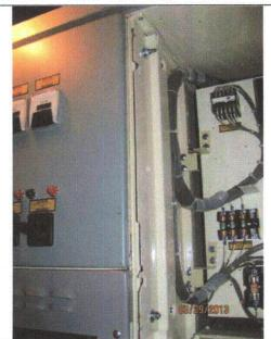
Note: Missing bolt holes identified connecting 1B4A with 69/1B4A.
