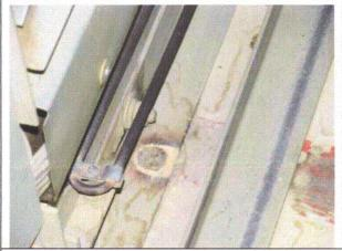
Note: Poor quality plug weld in 1A3-3.
