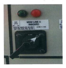
If the MAIN STEAM LINE A INBD ISOLATION VLV (MSIV) XFS switch, 2-XS-1-14, is placed in EMERG while 2-HS-1-14C handswitch is positioned as shown above, this MSIV will \_\_(1)\_\_.
