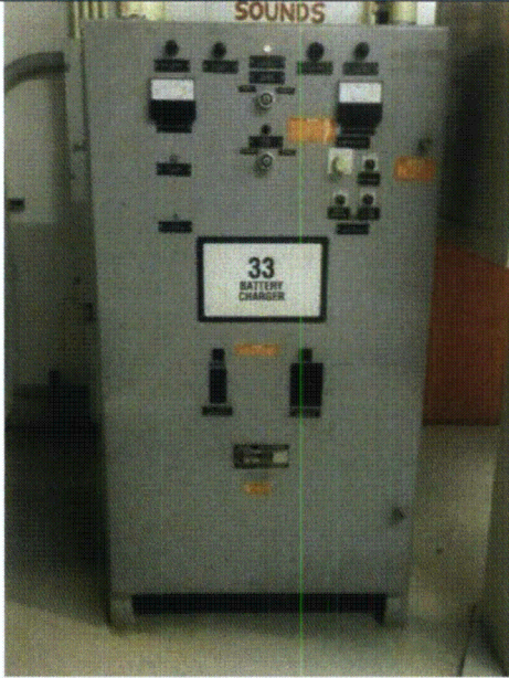
Note: Front View of BATT CHGR 33
