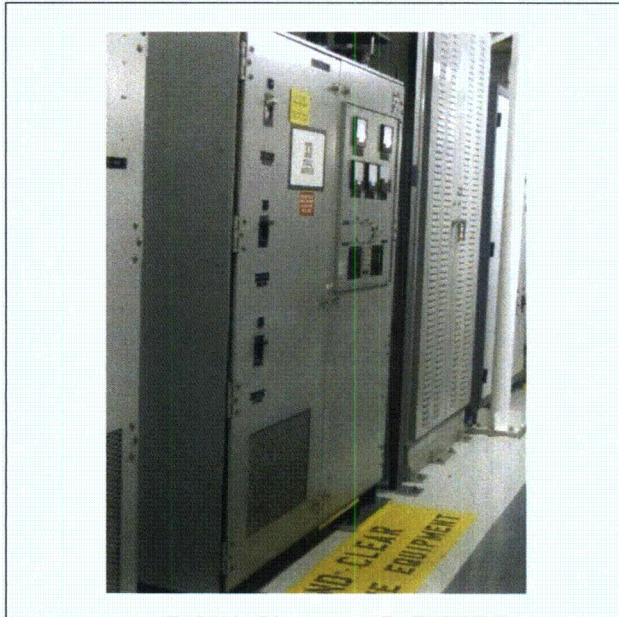
Note: STATIC INVERTER 33
