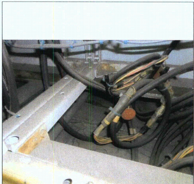
Housekeeping issue Tie wraps left inside the floor space
