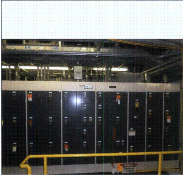
36AMCC anchorage and interior were inspected due to its similarity with 36BMCC
