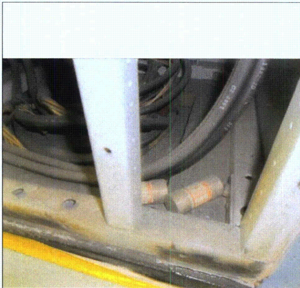
Housekeeping issue Fuse left inside the floor space
