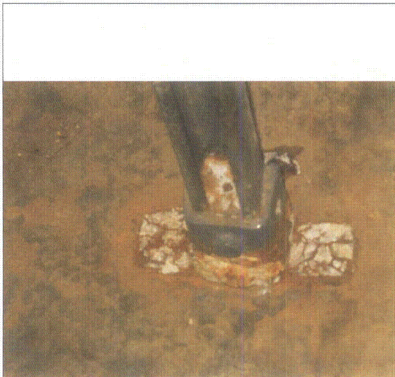
Note: Electric heat tracing cabinet base plate inside of curbed area.
