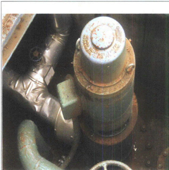
Note: F.O. Transfer Pump
