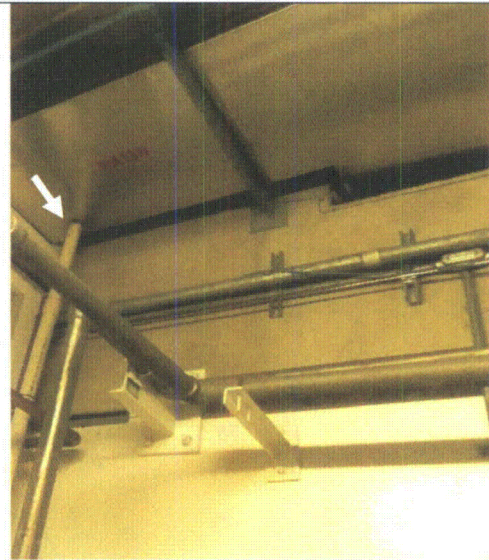
Note: PVC penetrates duct
