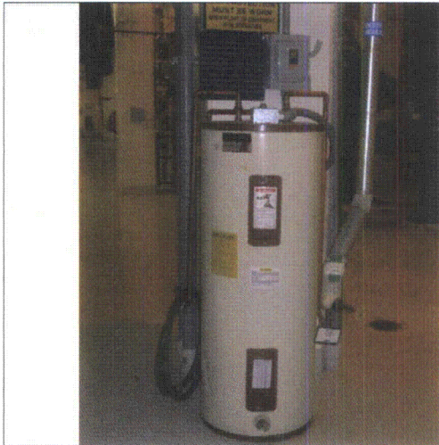
Note: Hot water heater with no apparent restraint
