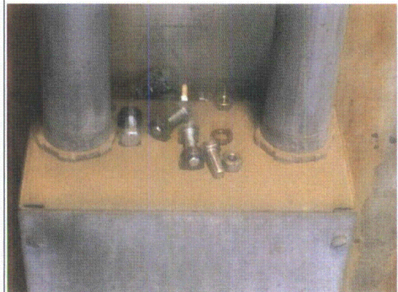
Note: Bolts and nuts on top of electrical box for GAI-Tronics.
