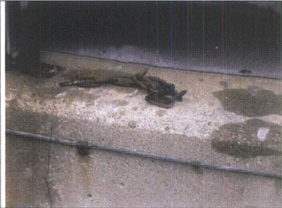
Note: Loose chain on top of RWST-31 foundation.
