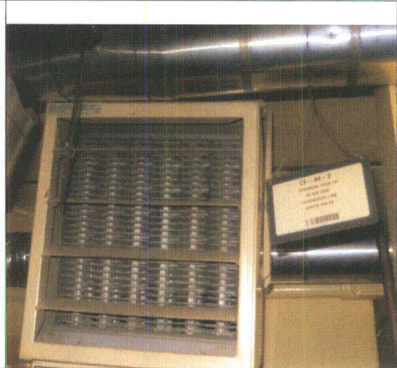
Note: Pipe insulation with heater.
