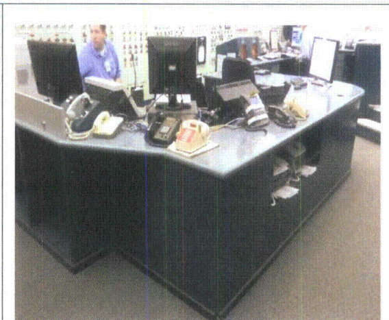
Note: Unrestrained phones, printers and monitors at work stations
