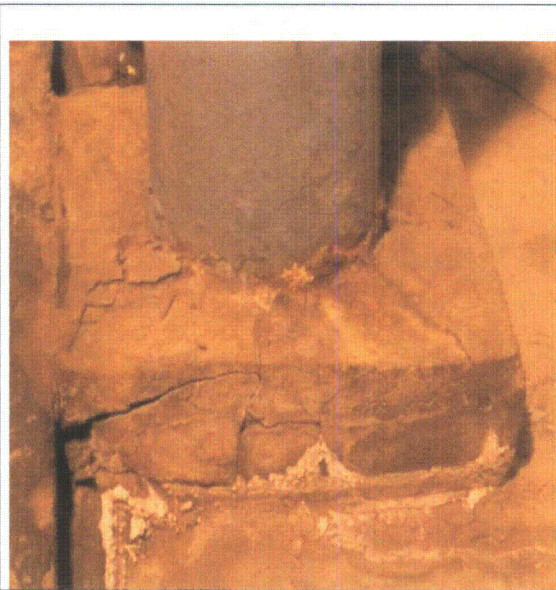
Note: Cracked grout penetration protection
