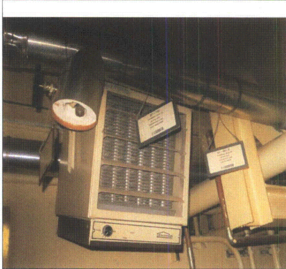
Note: Pipe insulation interference with heater.
