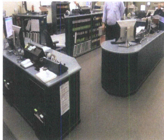
Note: Unrestrained phones, printers and monitors at work stations
