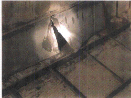
Note: Broken flashing
