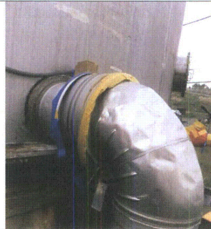
Note: Piping insulation connection held with tape.
