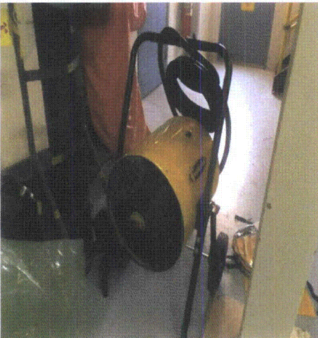
Note: An unrestrained heater and power supplier device on a wheeled cart
