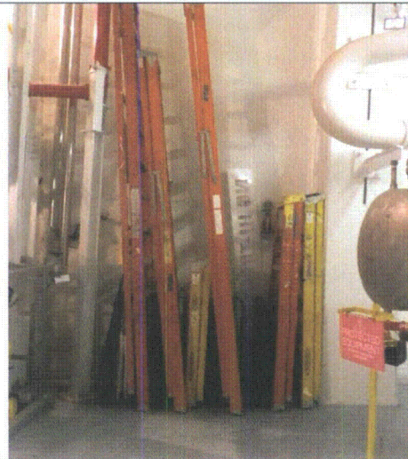
Note: Unrestrained ladders in a rack
