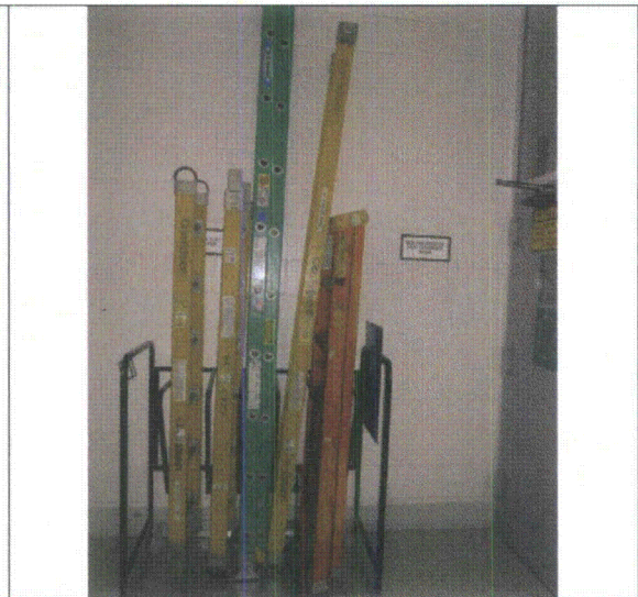
Note: Unsecured ladders at the Nonregenerative heat exchanger room
