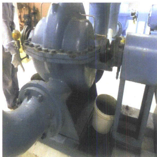
Note: Bucket at 32 CCW pump
