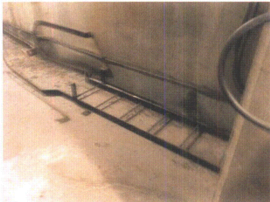
Note: unrestrained ladder by the north wall.
