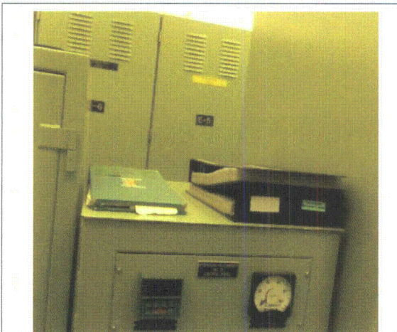
Note: unrestrained binders on top of Hydrogen Recombiner No. 31 Control Panel
