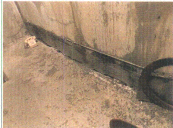
Note: Missing flashing along the wall
