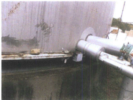
Note: Rock resting on the tank ring.
