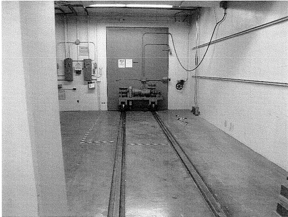
Figure 8, A010 Door in place
