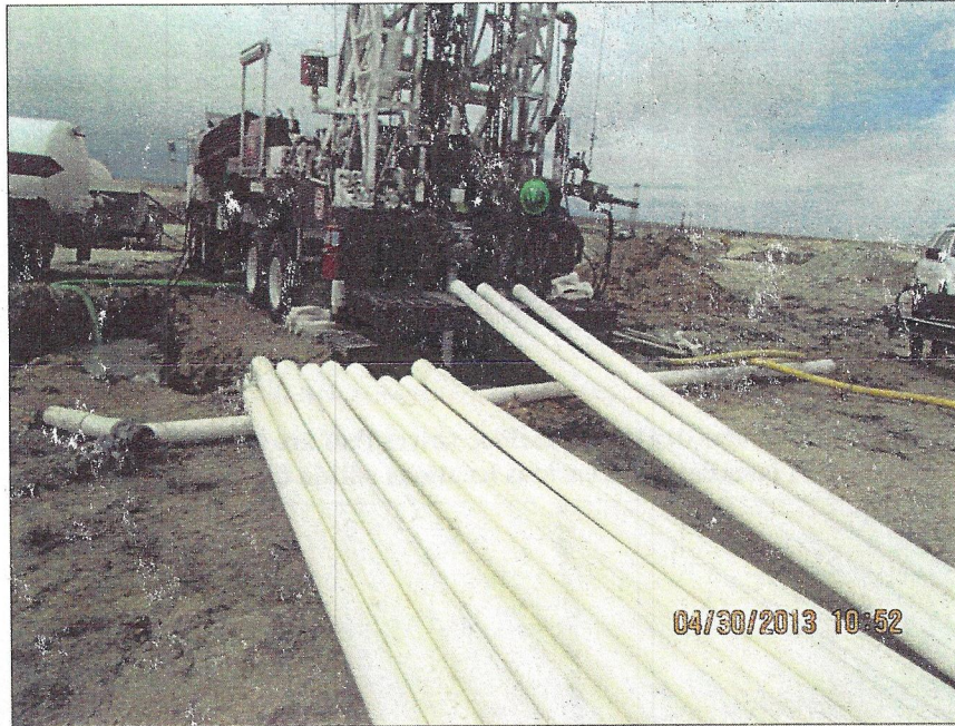
Photo Number 11: This depicts the 20-foot lengths of well casing that was staged behind one of the MU1 Pattern Area wells that was being cased today. The outer diameter of this casing is 4.95" and the inner diameter is 4.25".
