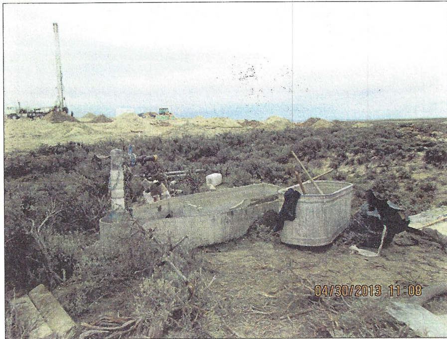
Photo Number 17: This depicts a portable mud-pit arrangement that was being used at one of the MU1 pattern area pilot holes that is located near an ephemeral drainage.
