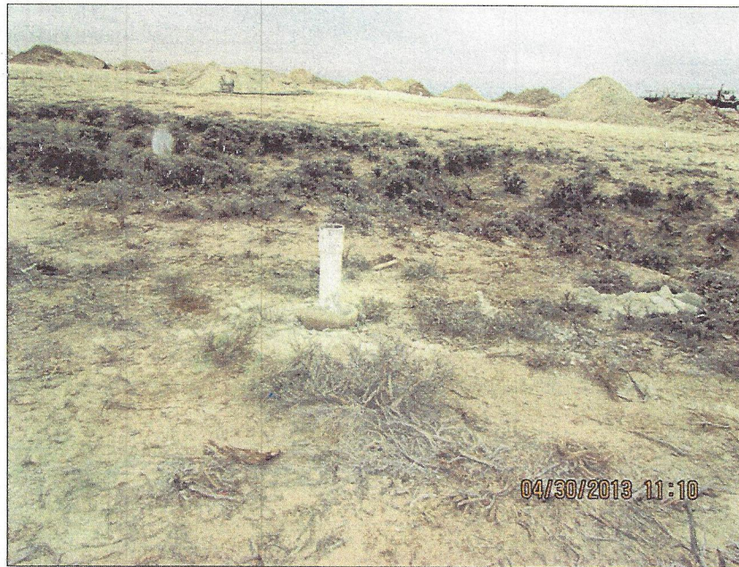
Photo Number 20: This depicts a cased well installed near an ephemeral drainage. The portable mud pit was used for this well's installation. The footprint of the affected area associated with this well is, not surprisingly, significantly smaller than wells drilled with in-ground mud-pits.
