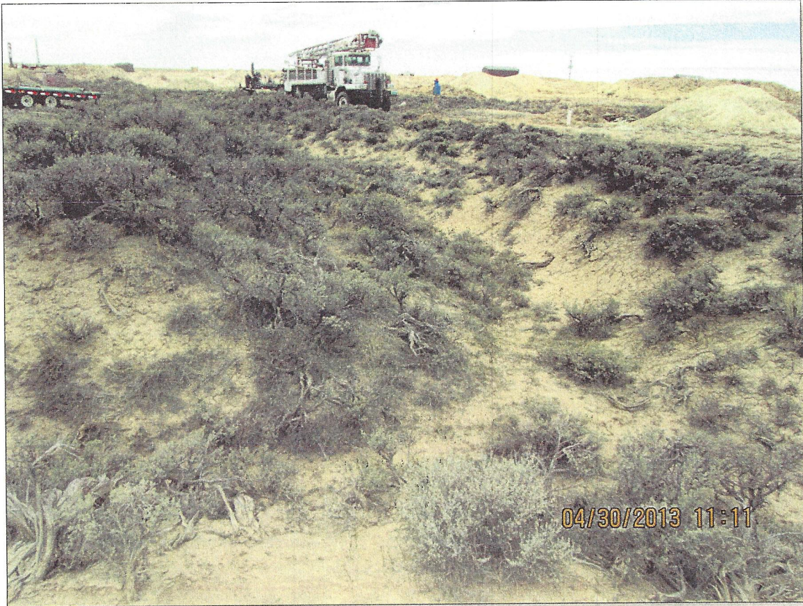
Photo Number 10: This is a view looking down-gradient at the ephemeral drainage near the well depicted in the above photo. The main purpose in using portable mud-pits is to prevent any spillage of drilling mud down the drainage. No drilling fluids were released into this drainage during the installation of the well depicted above in Photo Number 20.
