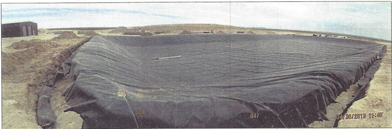
Photo Number 5: This depicts the bottom (geomembrane) liner that was recently installed in the north Pond. Its leak detection system has been installed and this pond will receive a layer of sand before the second liner is installed.
