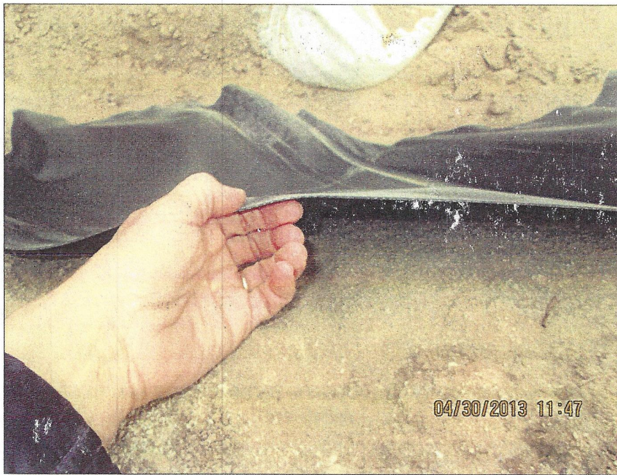
Photo Number 7: This a close-up view of the geomembrane liner material for the Ponds.
