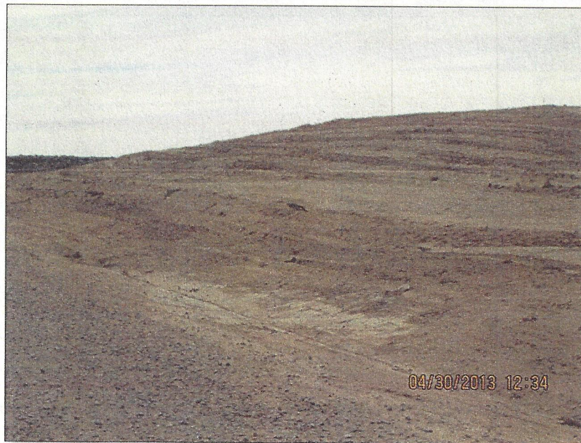
Photo Number 1: This depicts a topsoil stockpile along the west site access road that was recently seeded.
