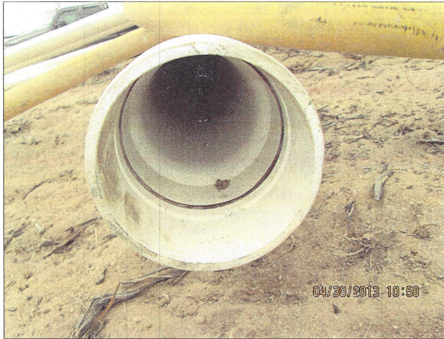
Photo Number 15: This depicts the bell end of one of the 20 foot sections of PVC well casing. The dark circle is an O-ring and part of the spline lock system. The groove in front of the black O-ring will receive the spline material (hard plastic “string”) once this casing is attached to the adjacent piece of casing.
