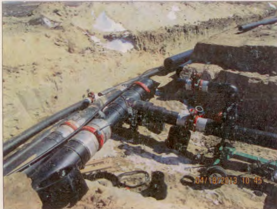
Photo Number 8: This depicts an intersection of the main trunkline (left) and a subsidiary pipe line trench to the MU1 Pattern Area.
