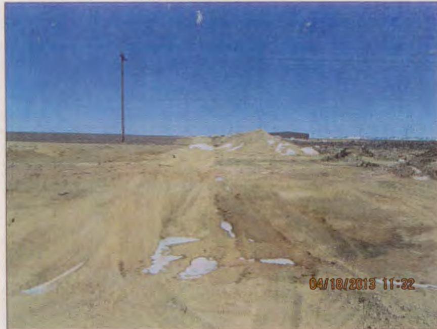
Photo Number 24: This is a view looking north at the main trunk line trench just north of where it goes under the site's access road. The trench was recently backfilled at this location. This photo can be compared with Photo Number 7 in the March 27, 2013 Inspection Report, which depicts the same trench when it was still open.
