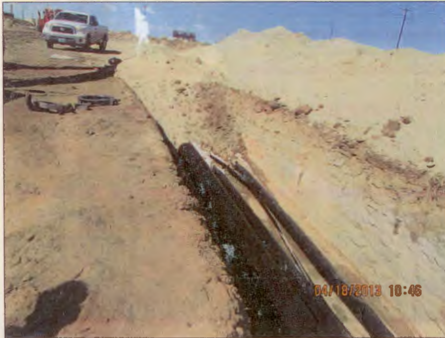
Photo Number 7: This depicts the main trunk line trench in the MU1 Pattern Area. The trench is in the process of being backfilled after pressure testing on Friday April 12, 2013 revealed the pipeline was sound.
