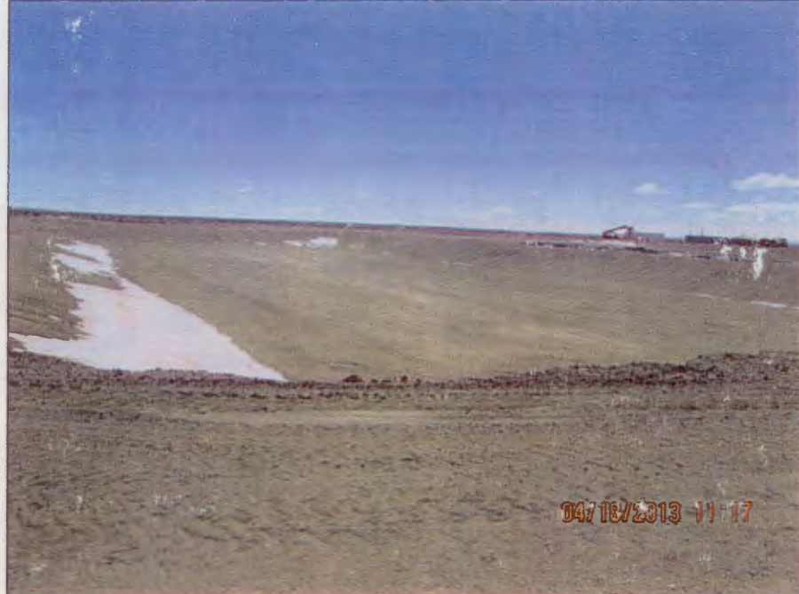
Photo Number 21: This depicts the northern pond just east of the Plant Building. Both ponds (north and south) were recently re-graded to clean up minor sloughing that had occurred over the winter. This view is looking east.
