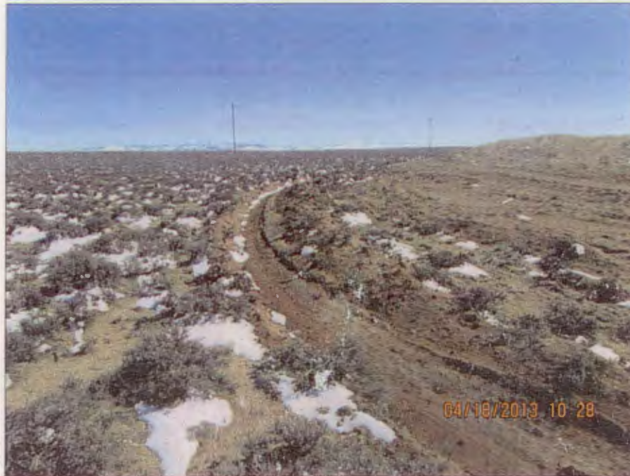
Photo Number 5: This is another view of the v-ditch around the base of topsoil stockpile 4. The v-ditch is well-constructed.
