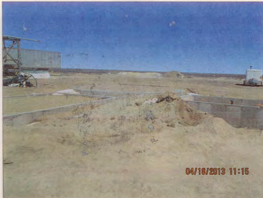
Photo Number 20: This depicts the footings for the 80,000 gallon tank that will be staged northwest of the Plant Building for fire suppression.
