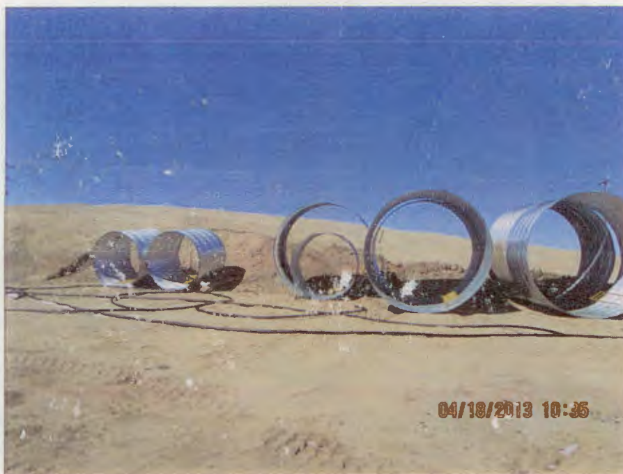
Photo Number 6: This depicts the large-diameter corrugated "culverts" that are being staged at the DDW-4 drill pad site before they are installed in the MU1 Pattern Area as "galleries" for housing manifolds.
