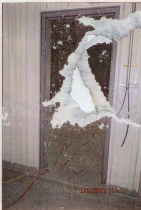
Photo Number 14: This depicts a doorway inside the Plant Building. Note the containment berm at the foot of the doorway. Every portion of the Plant Building is separated from the adjacent section with a containment berm.
