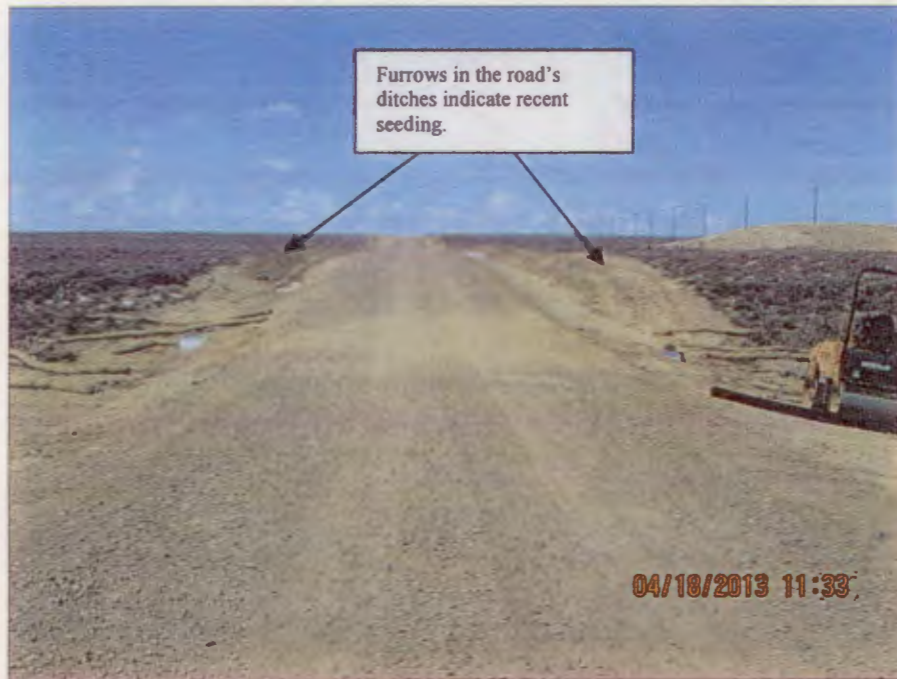
Photo Number 25: This depicts the site's access road west of the MU1 Pattern Area where LCI personnel have recently seeded the road's ditches. Note the disc furrows in the ditches. This view is looking west.
