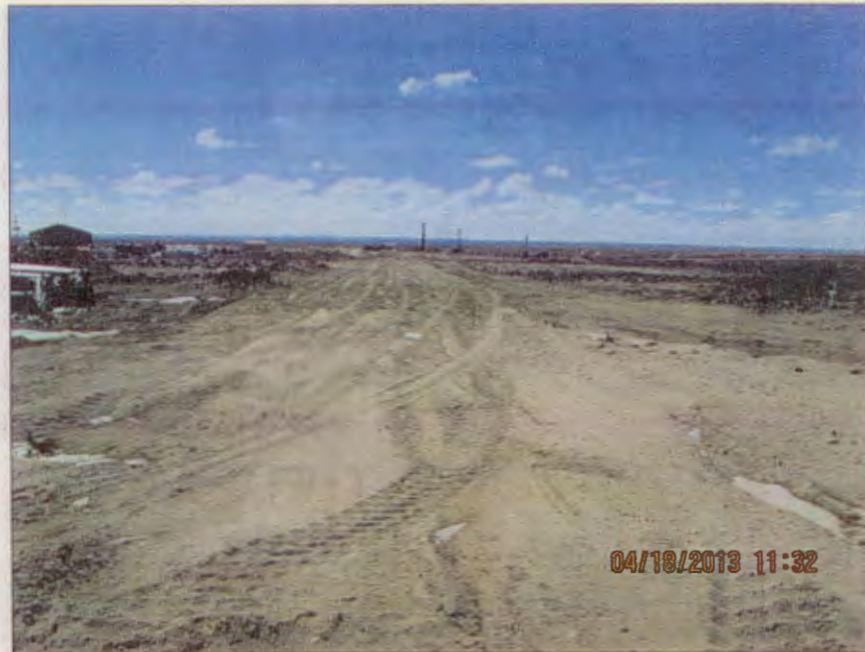
Photo Number 23: This is a view looking south at the main trunk line trench just south of where it goes under the site's access road. The trench was recently backfilled at this location. This photo can be compared with Photo Number 6 in the March 27, 2013 Inspection Report, which depicts the same trench when it was still open.
