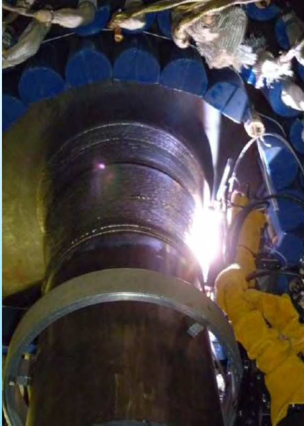
Weld overlay in progress
