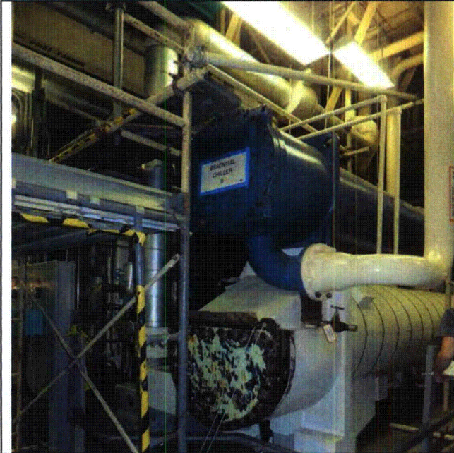
Note: Essential Chiller B
