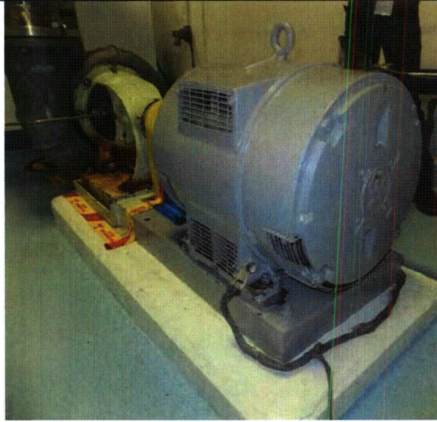
Note: Fuel Pool Pump B Motor
