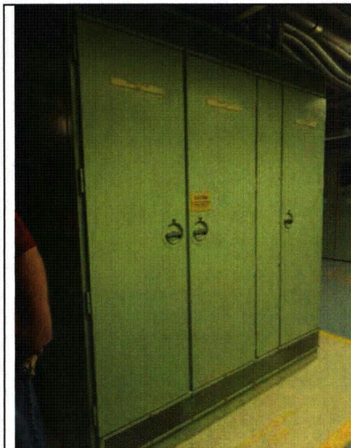
Note: Local Control Panel PAC LCP-61
