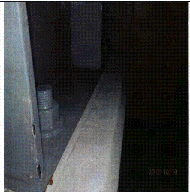
Note: Example of anchorage on Fuel Pool Heat Exchanger
