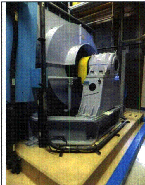
Note: Example of Emergency Diesel Generator B anchorage
