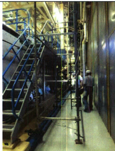
Note: Emergency Diesel Generator B
