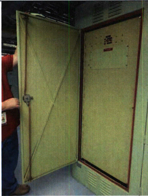
Note: ESFAS Cabinets
