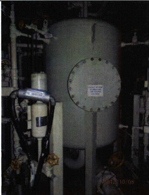
Note: Component Cooling Water Surge Tank
