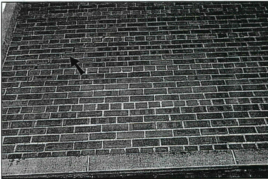
Figure A-4. Cracked southeast corner wall.
