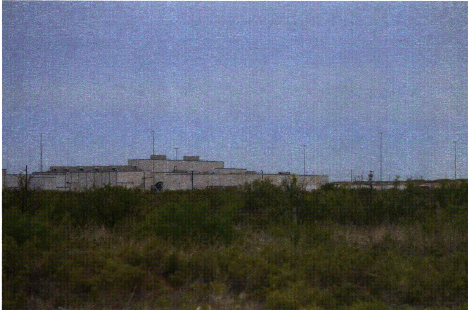
Figure 3.9-1C URENCO USA Facility as Seen From the West Looking East. (Photograph Taken 26 April 2012)
