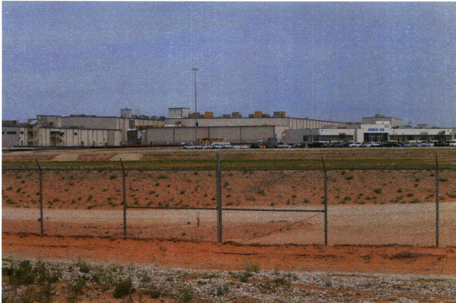
Figure 3.9-1A URENCO USA Facility as Seen From Highway 234/176, Looking North. (Photograph Taken 26 April 2012)
