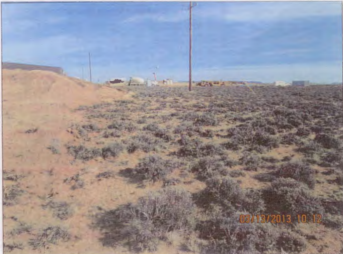
Photo Number 7: This depicts the south edge of the topsoil stockpile depicted in the photo above. In the foreground of this photo, topsoil from the stockpile can be seen on native ground. This speaks to the need to install toe ditches around the site's topsoil stockpiles.
