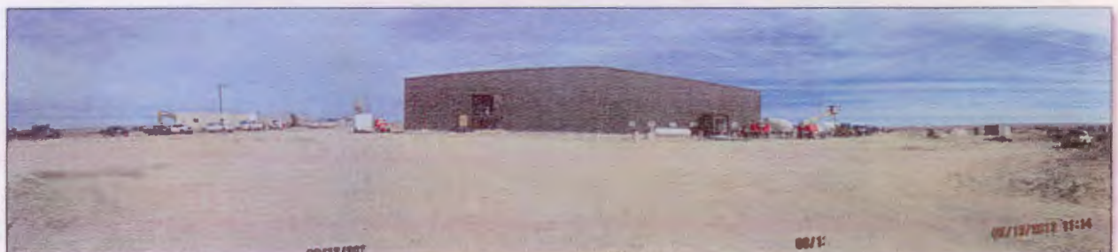
Photo Number 10: This is a panoramic looking toward the north at the south face of the Plant Building. This is the same vantage point as the majority of pictures of the Plant Site over the past several months.
