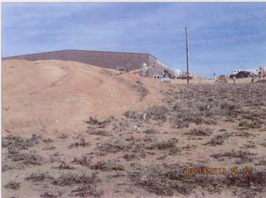
Photo Number 6: This is a view looking north along the east edge of the topsoil stockpile (TS-15?) that is directly across the road from the temporary office complex. It has early indications of topsoil sloughing onto native lands. A toe ditch is needed around this (and other) site topsoil stockpile(s).
