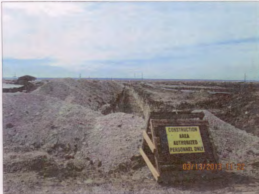
Photo Number 3: This depicts the northern extent of the main trunk line trench, where it meets the access road. View is looking south.
