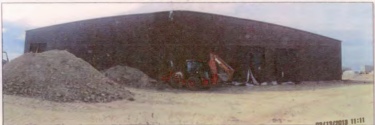
Photo Number 8: This panoramic depict the north side of the Plant Building. The view is looking to the south.
