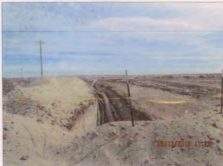
Photo Number 4: This depicts the portion of the main trunk line trench immediately north of the MU1 Pattern Area, where pipes were being laid. View is looking to the east.
