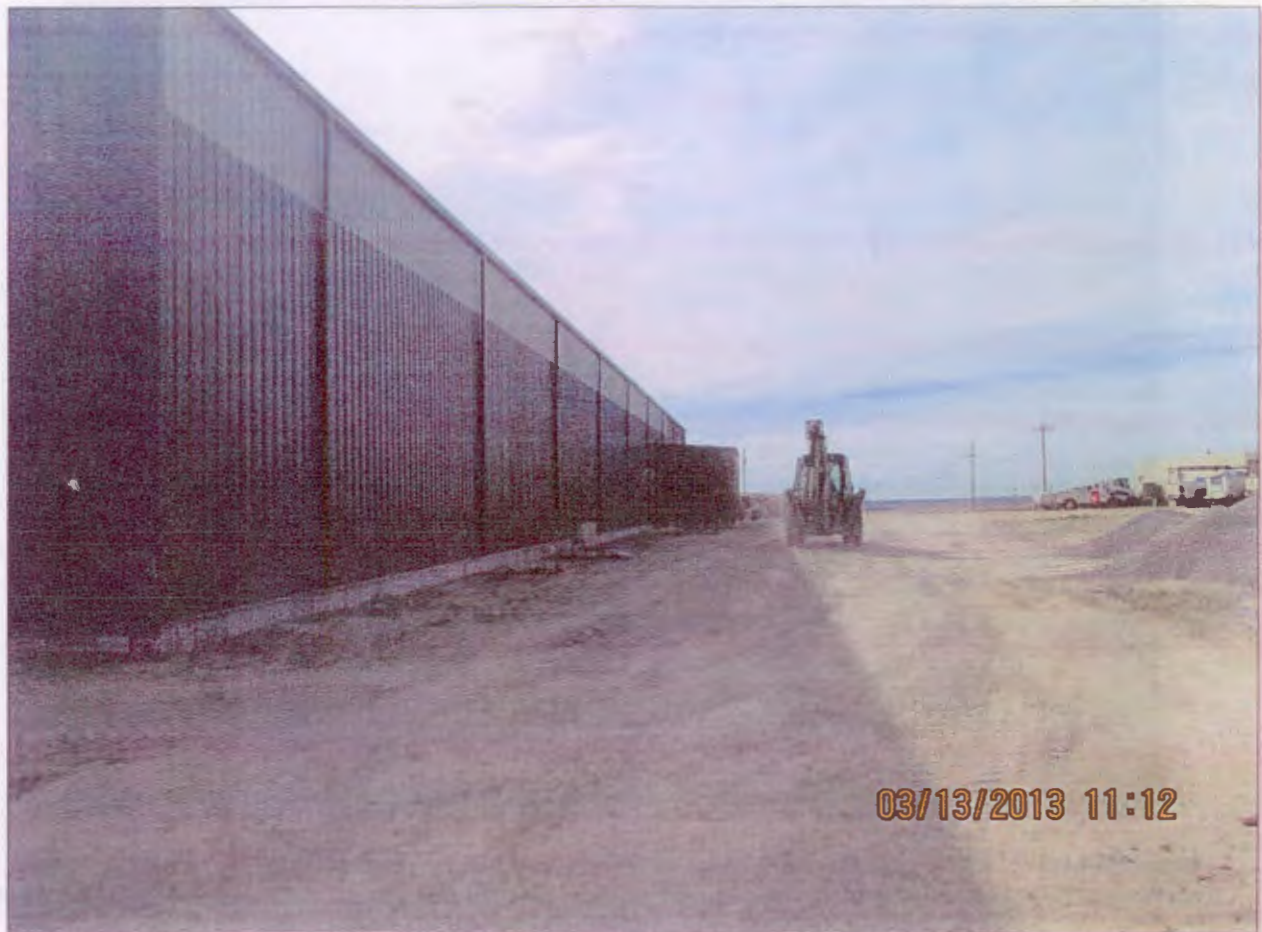
Photo Number 9: This is a view looking south along the west side of the Plant Building.
