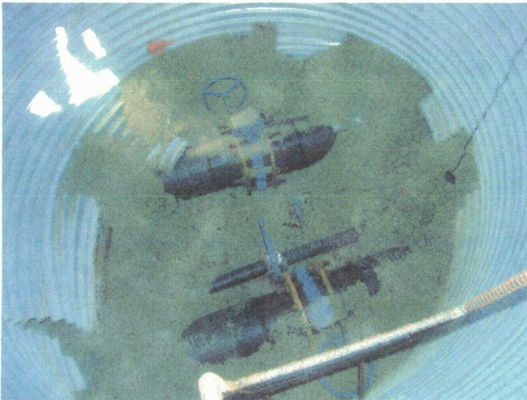
Figure 10 Replaced pipe with HDPE in Bellhole 41.
