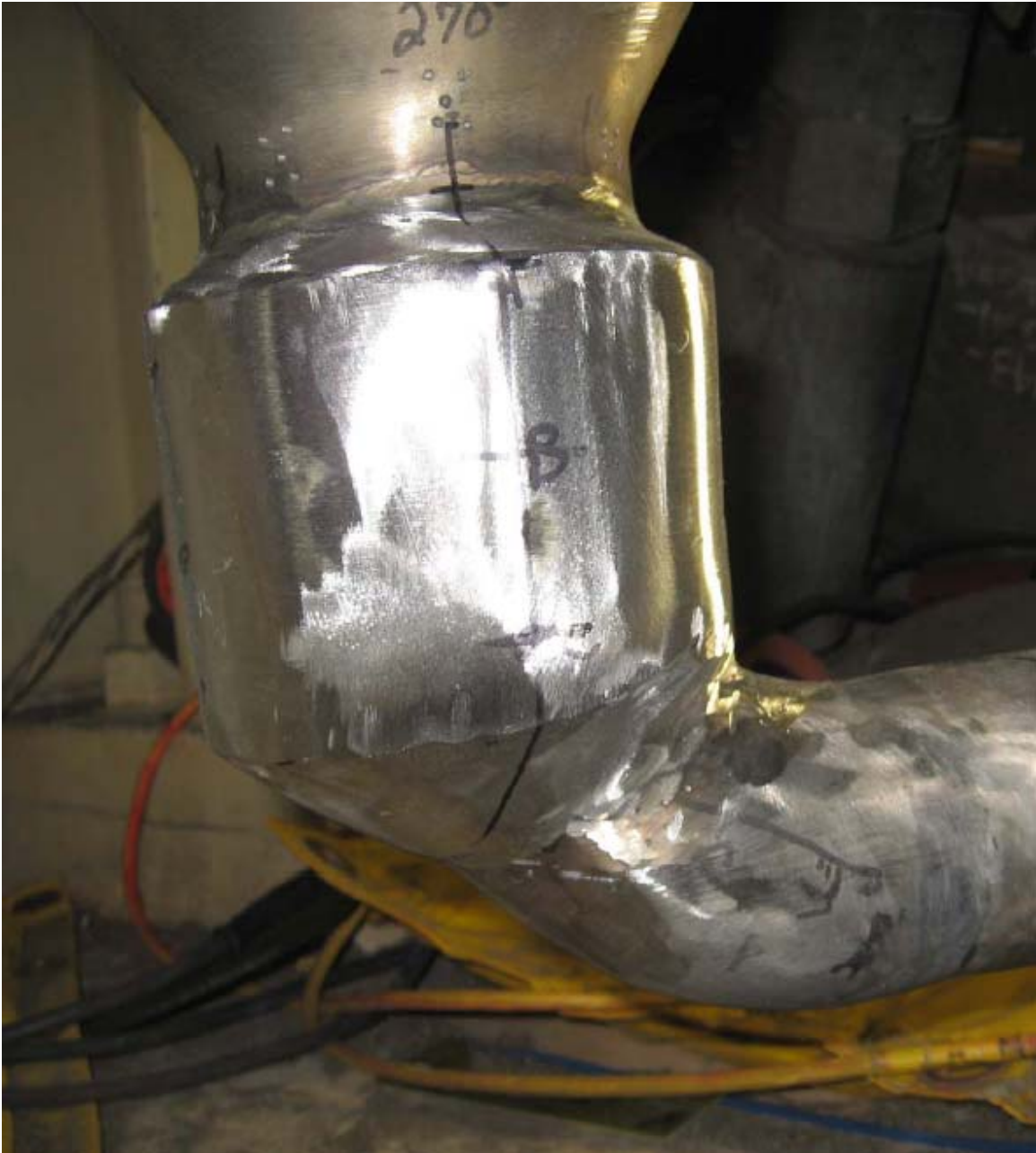
Image of Completed Full Structural Weld Overlay (FSWOL) [Weld RC-40-CCA-18-3-FW9]
