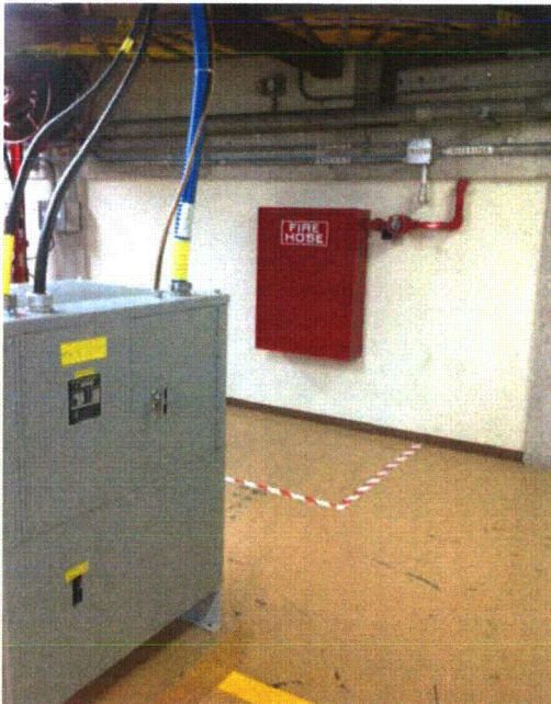
File Name: 1-67-3-1-06.jpeg Description: Fire protection valve near transformer judged to be adequately supported
