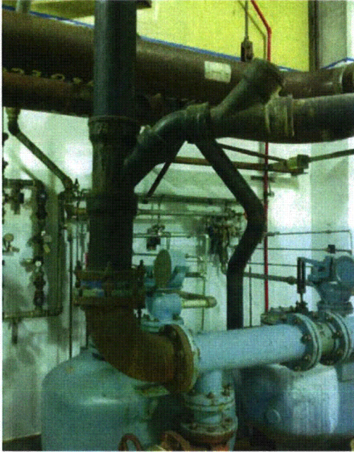
File Name: 1-71-1-1-01.jpeg Description: Cast iron pipe
