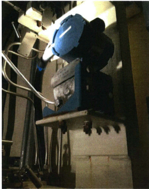
File Name: 1-68-1-1-12.jpeg Description: Surface corrosion identified
