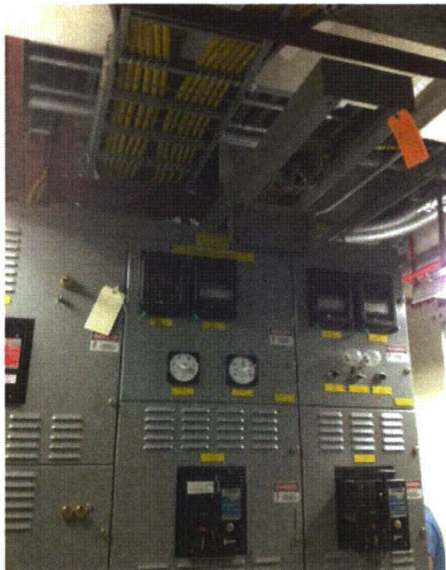
File Name: 1-60-3-1-02.jpeg Description: View of trolley on top of Cabinet
