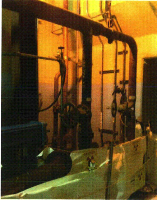
File Name: 1-68-3-1-18.jpeg Description: Rod Hung Sump Pump Piping
