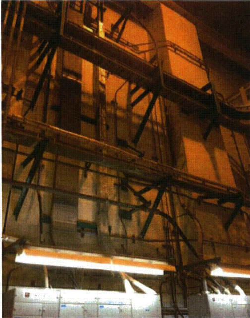
File Name: 1-59-1-1-05.jpeg Description: Raceways rigidly supported
