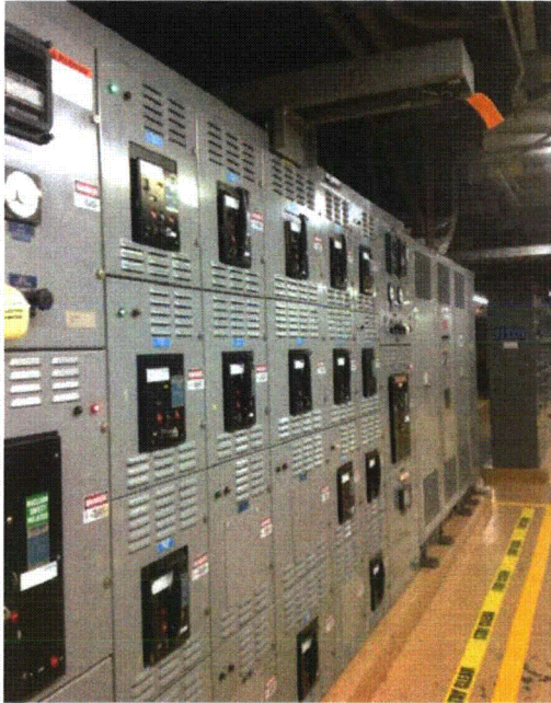
File Name: 1-74-1-1-06.jpeg Description: View of trolley on top of Cabinet
