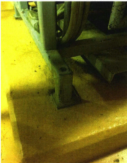
File Name: 1-74-1-1-01.jpeg Description: Air dryer rack (1P52-D003B) missing anchorage (similar issue 1P52-D003A)
