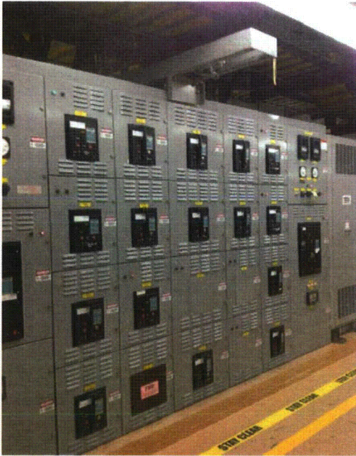
File Name: 1-71-3-1-06.jpeg Description: View of trolley on top of Cabinet
