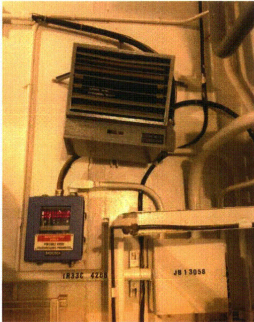
File Name: 1-65-1-1-08.jpeg Description: View of crooked heater. Not a concern for operability.
