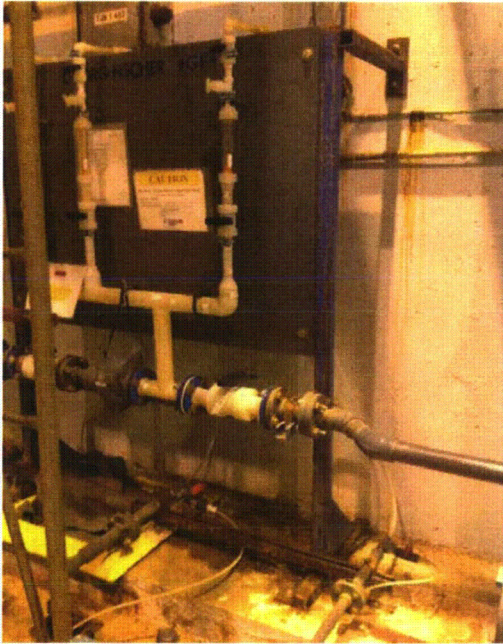
File Name: 1-70-1-1-05.jpeg Description: Surface corrosion identified
