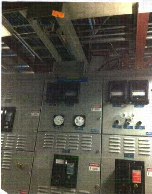
File Name: 1-66-1-1-02.jpeg Description: View of trolley on top of Cabinet
