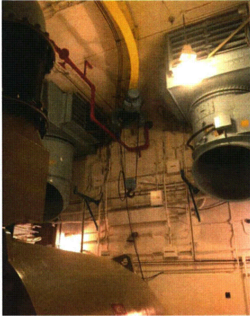
File Name: 1-65-2-1-08.jpeg Description: Crane away from components
