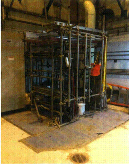
File Name: 1-67-1-1-05.jpeg Description: Scaffolding staging area
