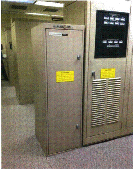
File Name: 1-67-1-1-03.jpeg Description: Cabinet not anchored
