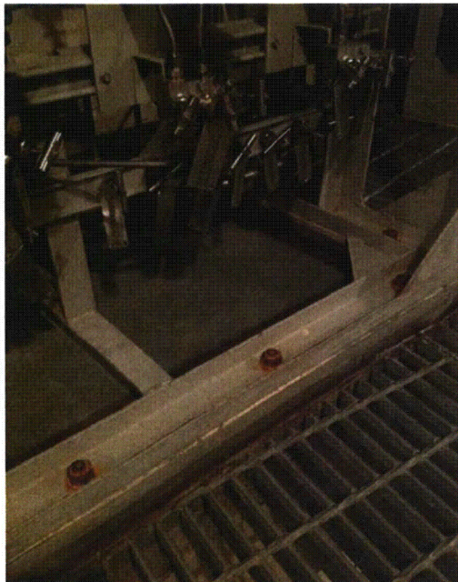
File Name: 1-65-1-1-13.jpeg Description: Corrosion in instrument rack anchorage
