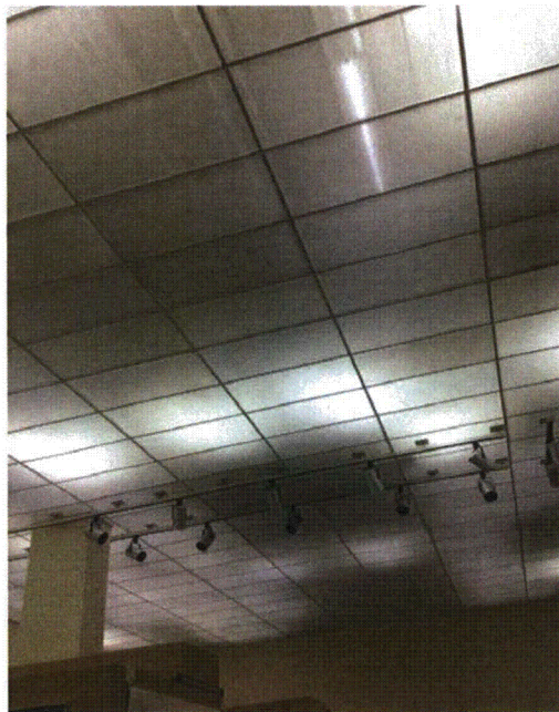
File Name: 1-60-1-1-03.jpeg Description: Ceiling tiles not anchored
