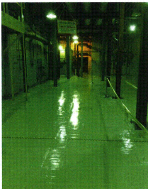
File Name: 1-66-3-1-18.jpeg Description: General view west hallway
