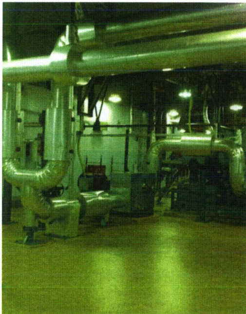
File Name: 1-60-1-1-01.jpeg Description: General view of room
