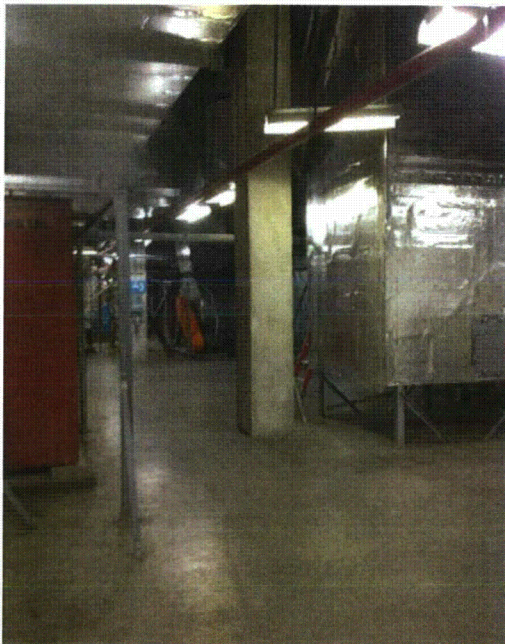
File Name: 1-59-1-1-04.jpeg Description: General view
