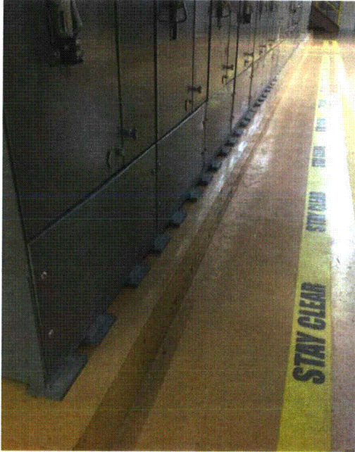
File Name: 1-68-1-1-06.jpeg Description: View of MCC EF1C07 anchorage (1R24-S0023)
