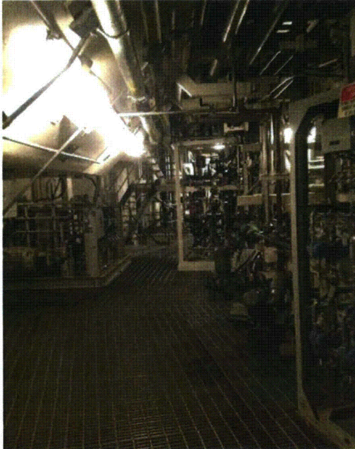
File Name: 1-59-1-1-13.jpeg Description: General view
