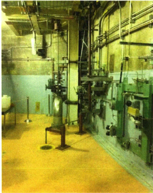
File Name: 1-59-2-1-16.jpeg Description: General view of room
