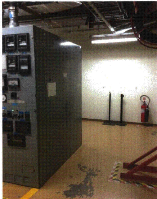
File Name: 1-72-1-1-06.jpeg Description: View of area where tool locker was located
