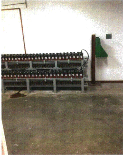
File Name: 1-59-1-1-07.jpeg Description: General view
