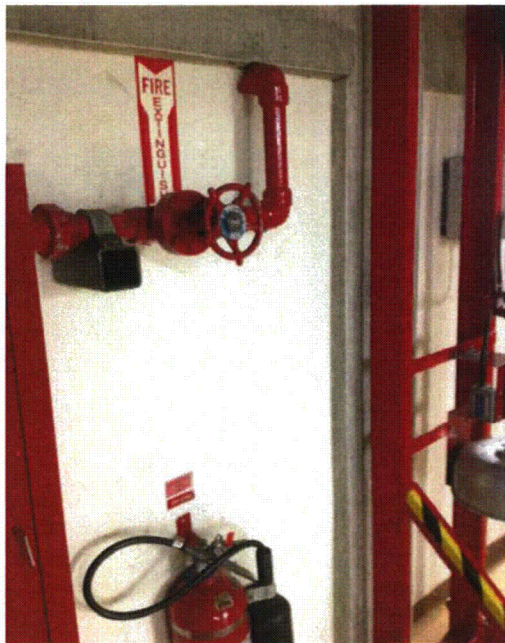
File Name: 1-65-1-1-06.jpeg Description: Fire protection valve well supported
