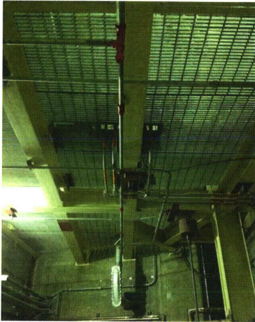
File Name: 1-65-2-1-16.jpeg Description: View of fire protection piping and overhead grating
