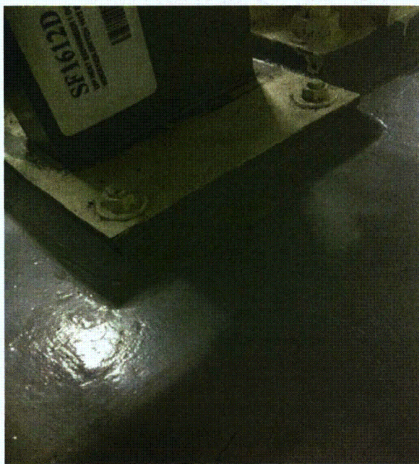
FIS1612 anchorage View of anchorage
