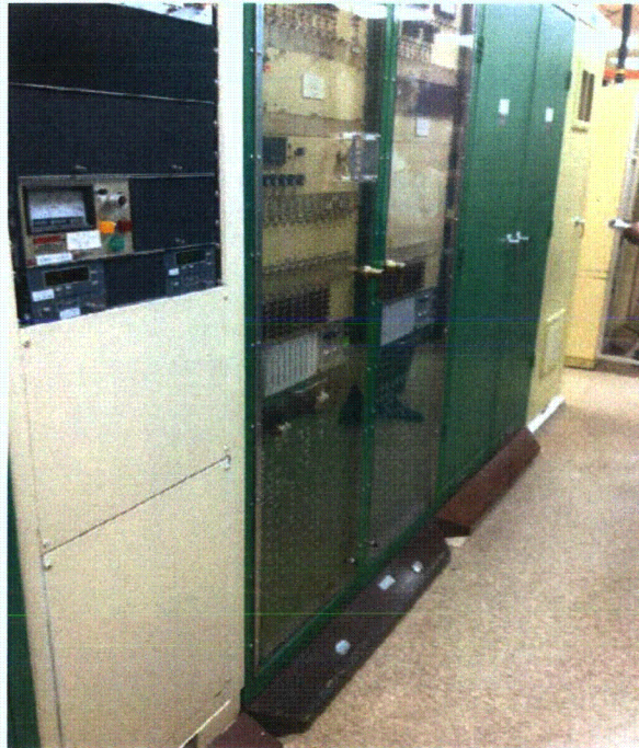
L311-511 cabinet General View of Cabinet housing components
