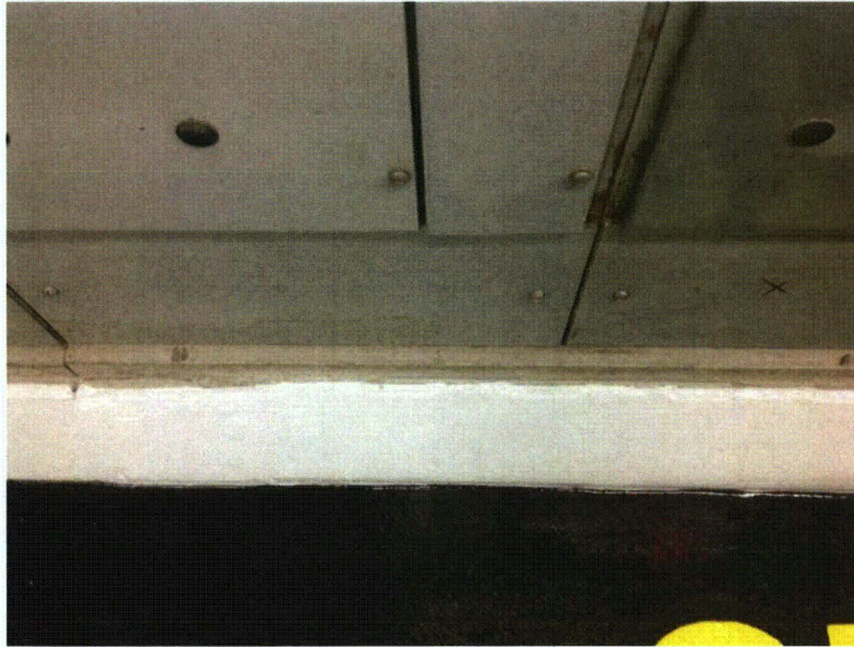
F12A stitch weld Partial view of anchorage, view is typical of all anchors
