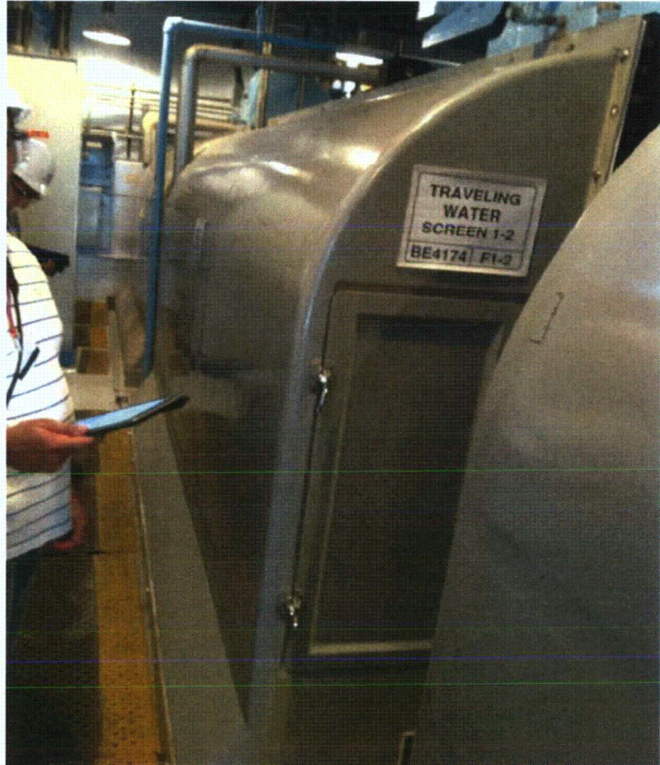
F1-2 general General view of component
