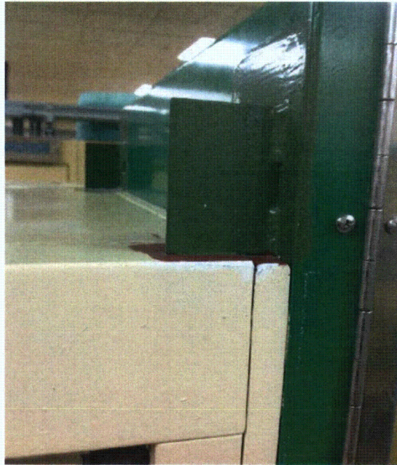
L311-511 cabinets welded together on left Cabinets are welded together on the left side
