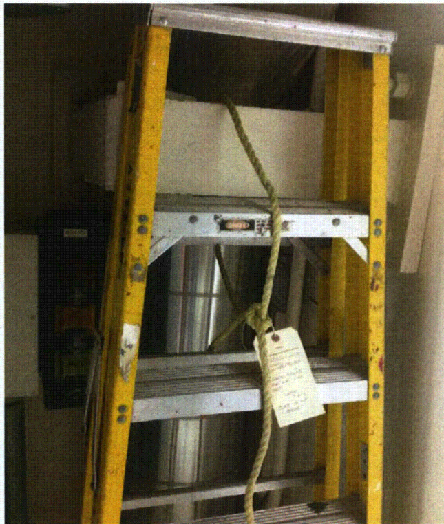
F11A poorly secured ladder in area of MCC Ladder loosely tied off.
