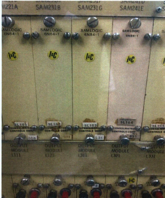
L311 General view of component
