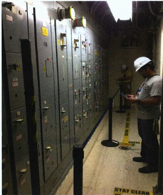
F11A general General view of component
