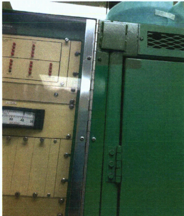
L311-511 cabinets welded together on right Cabinets are welded together on the right side
