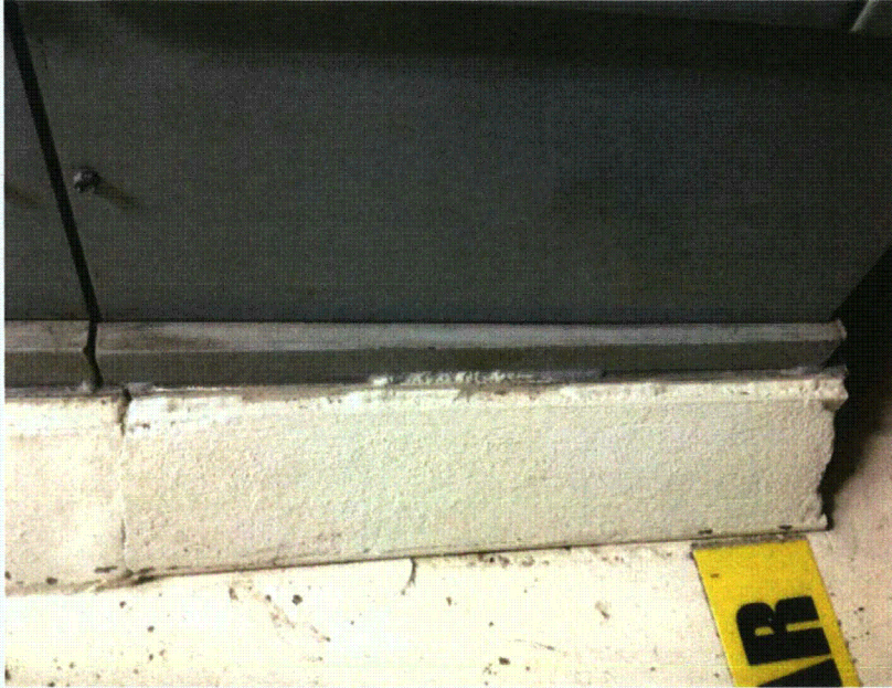
F11A crack in base of grout on corner Separation in base grout. Appears to be aesthetic grout only.
