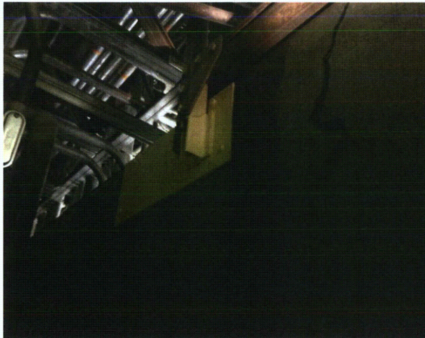
F11A rigid connection to adjoining conduit and MCC A rigid connection is used to fasten the unit to adjoining conduit
