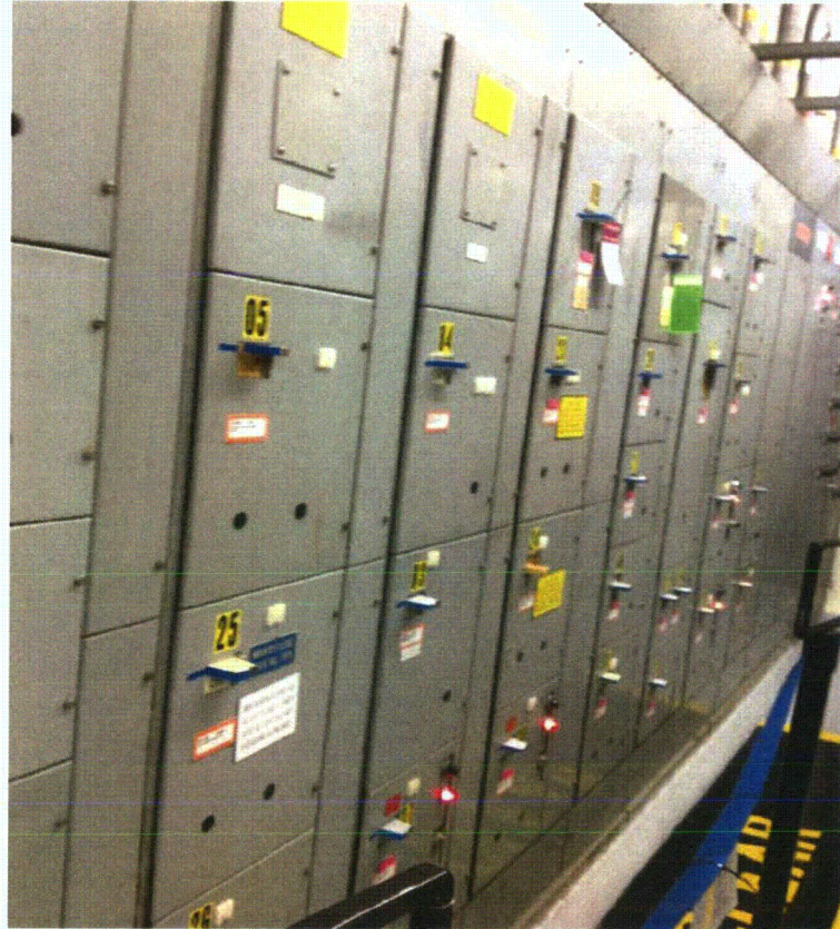
F12A general General view of component
