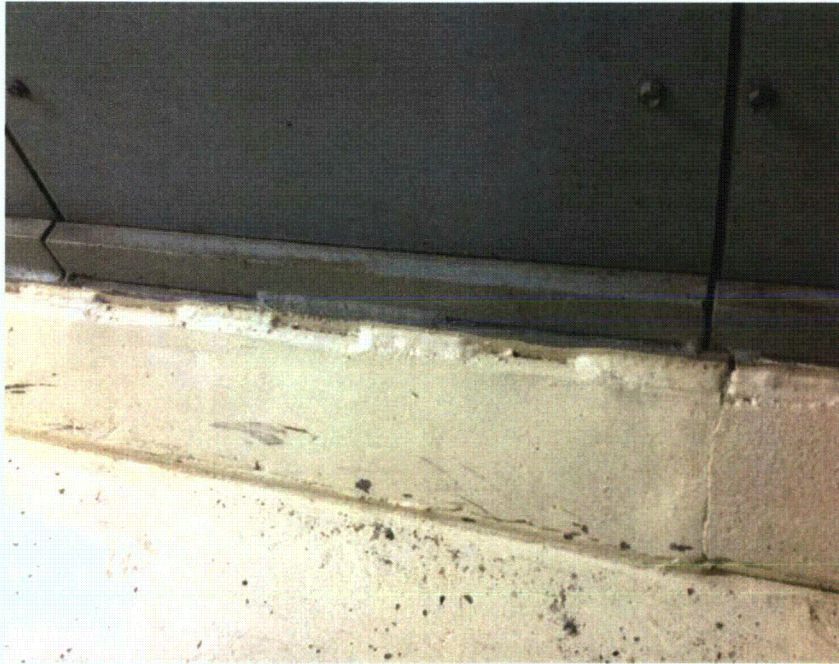
F11A stitch weld Partial view of anchorage, view is typical of all anchors
