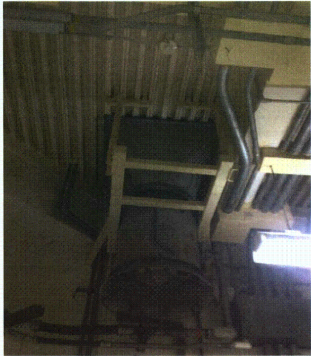
FD1062 anchorage View of anchorage
