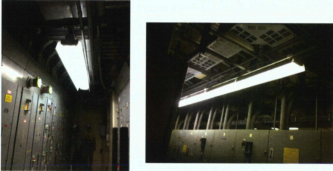
Figure 6-1: Unprotected Fluorescent Light Tubes
