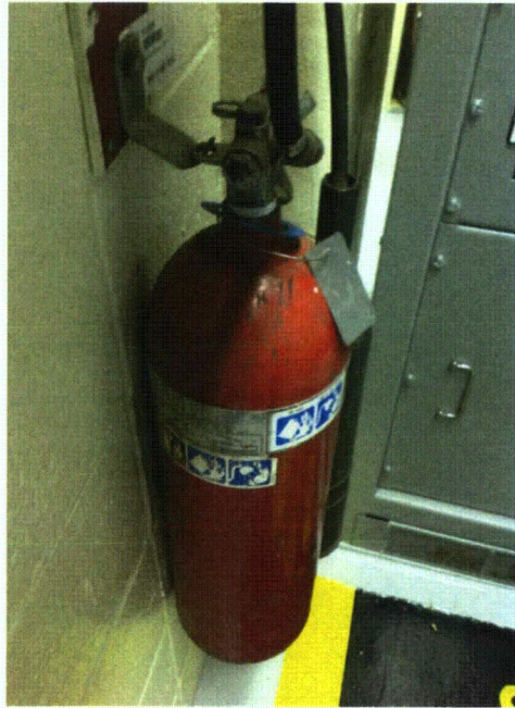
Figure 6-5: Typical Wall Mounting for Fire Extinguishers
