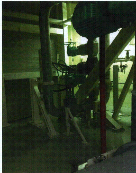
Figure 6-4: Support Conditions for Component CS1530
