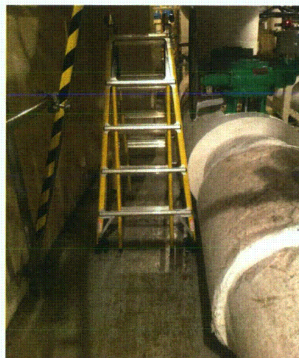
Figure 6-6: Unrestrained Maintenance Equipment
