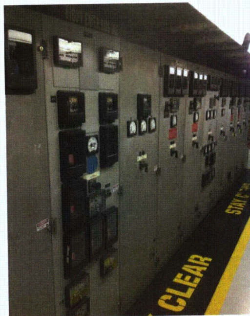
File Name: 2-64-9-1-25.jpeg Description: General view of component
