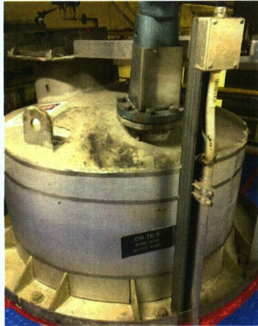
File Name: 2-63-6-1-60.jpeg Description: View of agitator mounting on Boric Acid Batch Tank
