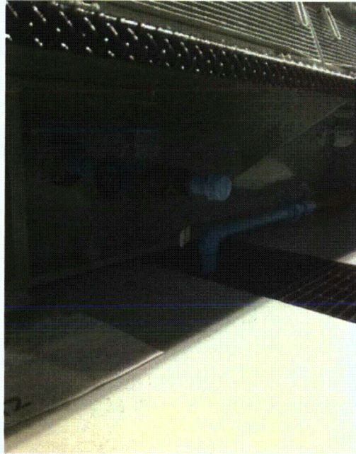
File Name: 2-73-8-1-20.jpeg Description: View of base detail showing no grout below DG's middle section.
