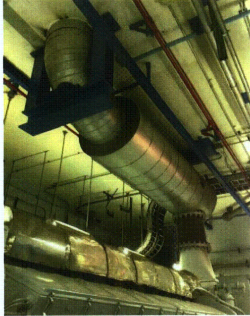
File Name: 2-63-8-1-20.jpeg Description: View of marks surrounding DG exhaust pipe.
