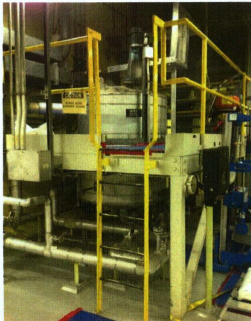
File Name: 2-64-6-1-60.jpeg Description: View of platform surrounding Boric Acid Batch Tank
