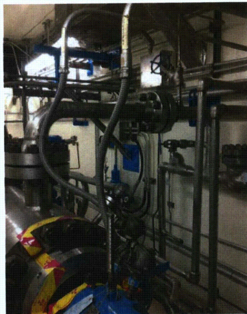
File Name: 2-73-1-1-17.jpeg Description: View of flexible attached lines
