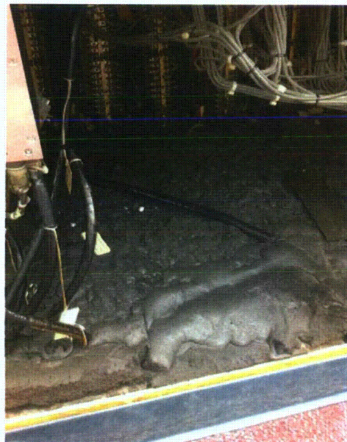
File Name: 2-62-5-1-18.jpeg Description: View of insulating material covering component anchorage
