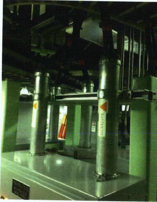
File Name: 2-73-1-1-60.jpeg Description: View of top entry conduits
