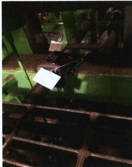
File Name: 2-62-5-1-60.jpeg Description: General view of component
