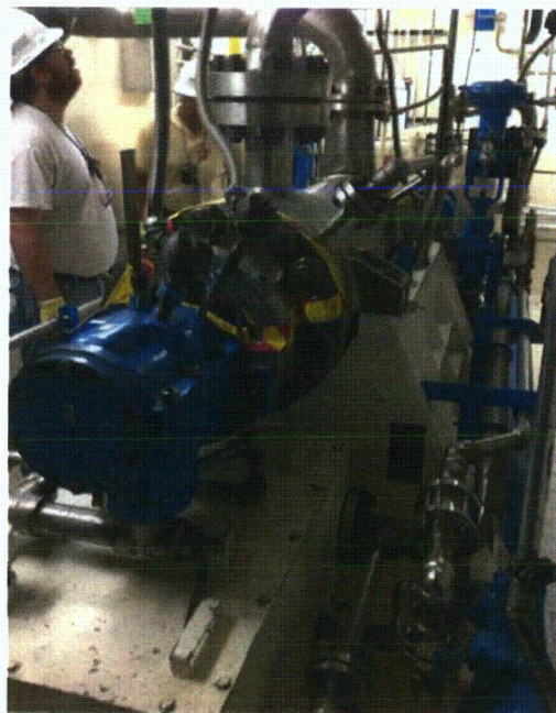
File Name: 2-62-1-1-17.jpeg Description: General view of component
