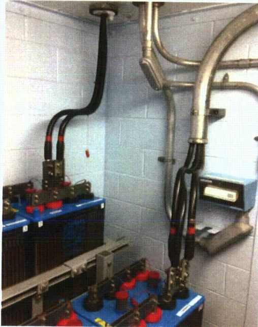
File Name: 2-62-1-1-11.jpeg Description: View of flexible attached lines
