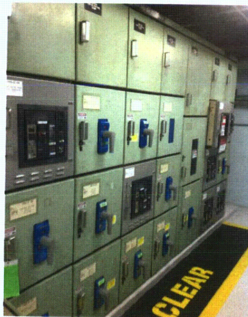
File Name: 2-62-4-1-26.jpeg Description: General view of component
