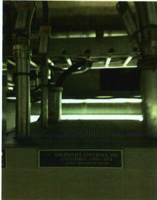
File Name: 2-63-1-1-02.jpeg Description: View of top entry conduits
