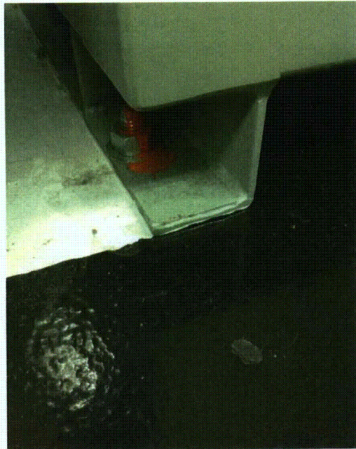
File Name: 2-73-1-1-02.jpeg Description: Close up view of component anchorage
