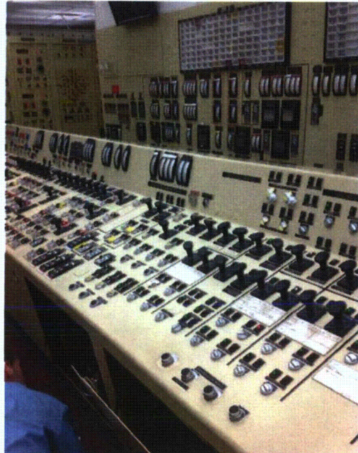
File Name: 2-61-5-1-18.jpeg Description: General view of component
