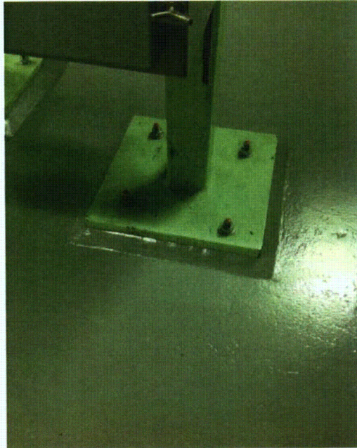
File Name: 2-63-1-1-60.jpeg Description: View of panel anchorage
