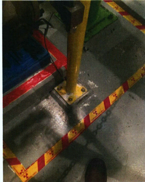
File Name: 2-63-4-1-60.jpeg Description: Anchorage detail for post base plate
