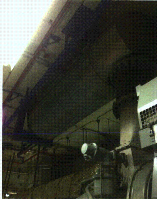
File Name: 2-63-3-1-21.jpeg Description: General view of DG exhaust pipe
