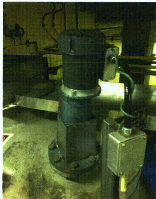
File Name: 2-62-6-1-60.jpeg Description: General view of component
