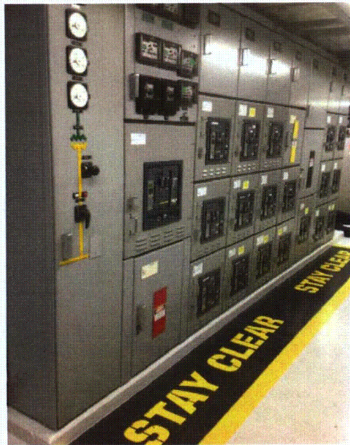
File Name: 2-62-10-1-25.jpeg Description: General view of component
