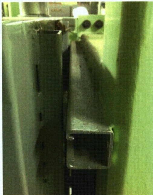
File Name: 2-64-1-1-60.jpeg Description: View of channel struts attached to posts
