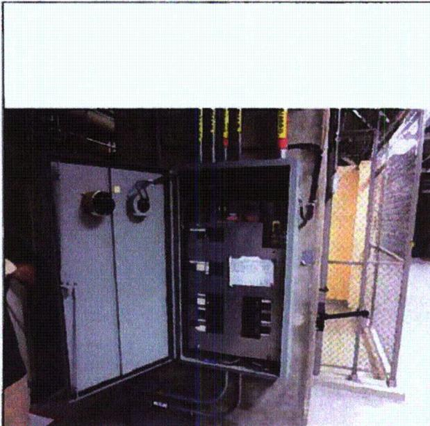
**Note:** Cabinet opened 10/11/12 and re-inspection completed. One nut not engaged for 50% of thread. No seismic concerns since 3 nuts are fully engaged.
