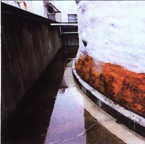
**Note:** *Condensate Storage Tank – Anchorage covered by insulation. No visible cracks around the tank foundation*
