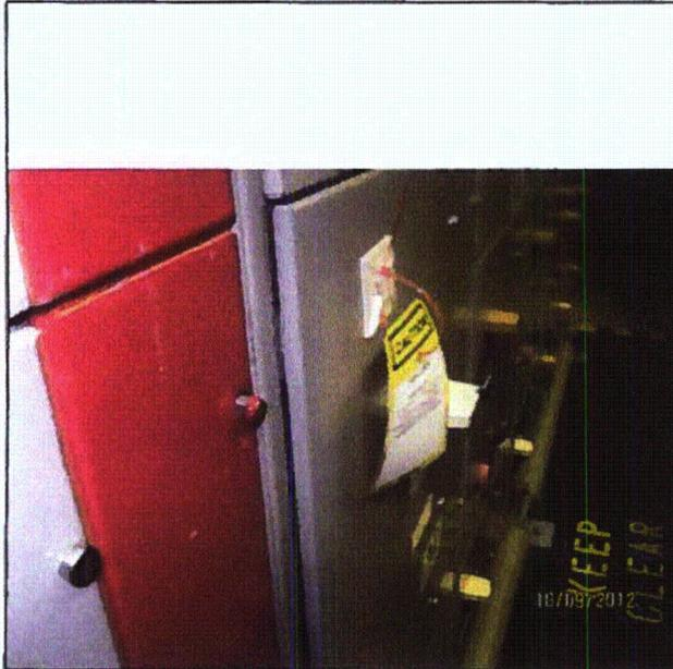
**Note:** *Loose bolts at connection of MCC8 and MCC7*
